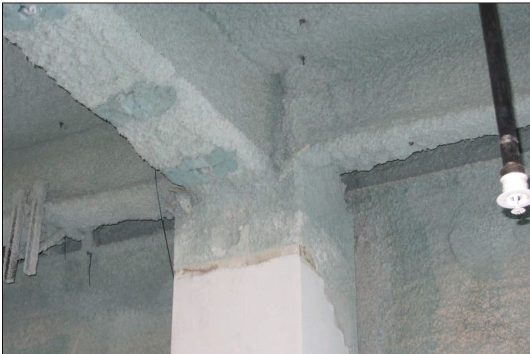
Photo 4 – Typical Beam to Column Connection
