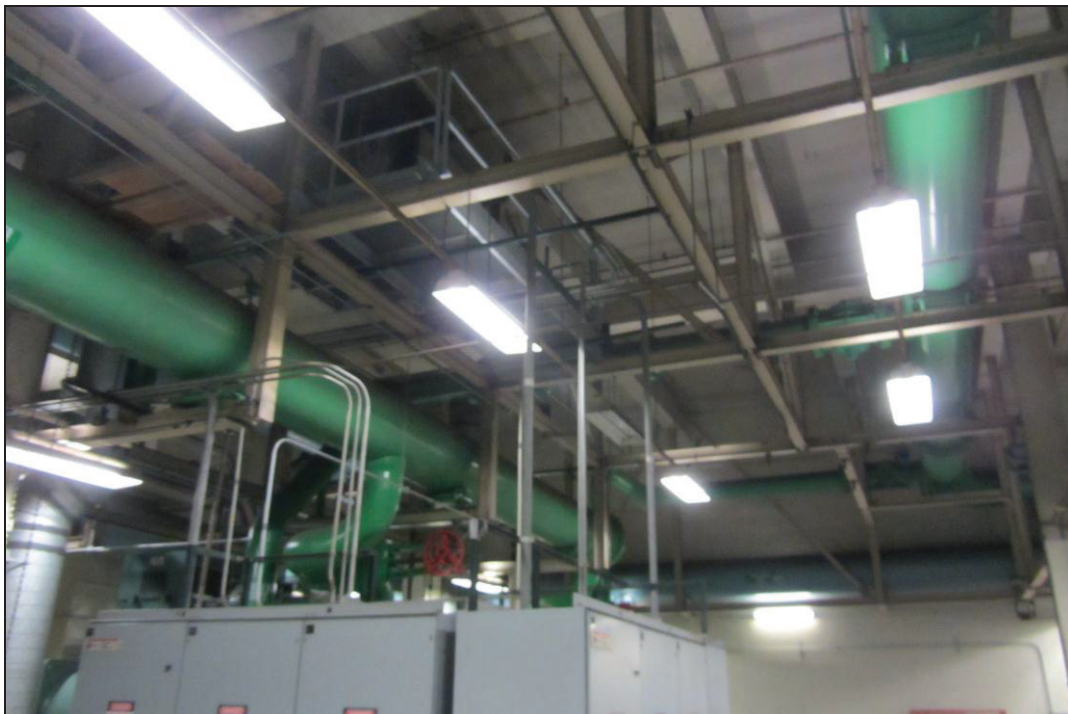
Photo 6 – Bracing of Piping System
