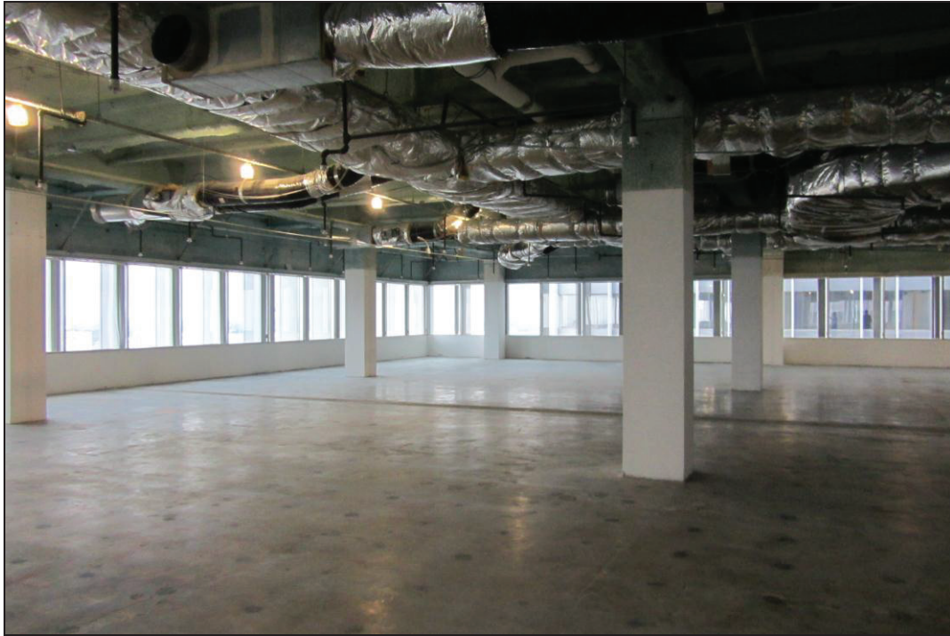
Photo 3 – Typical Steel Framing
