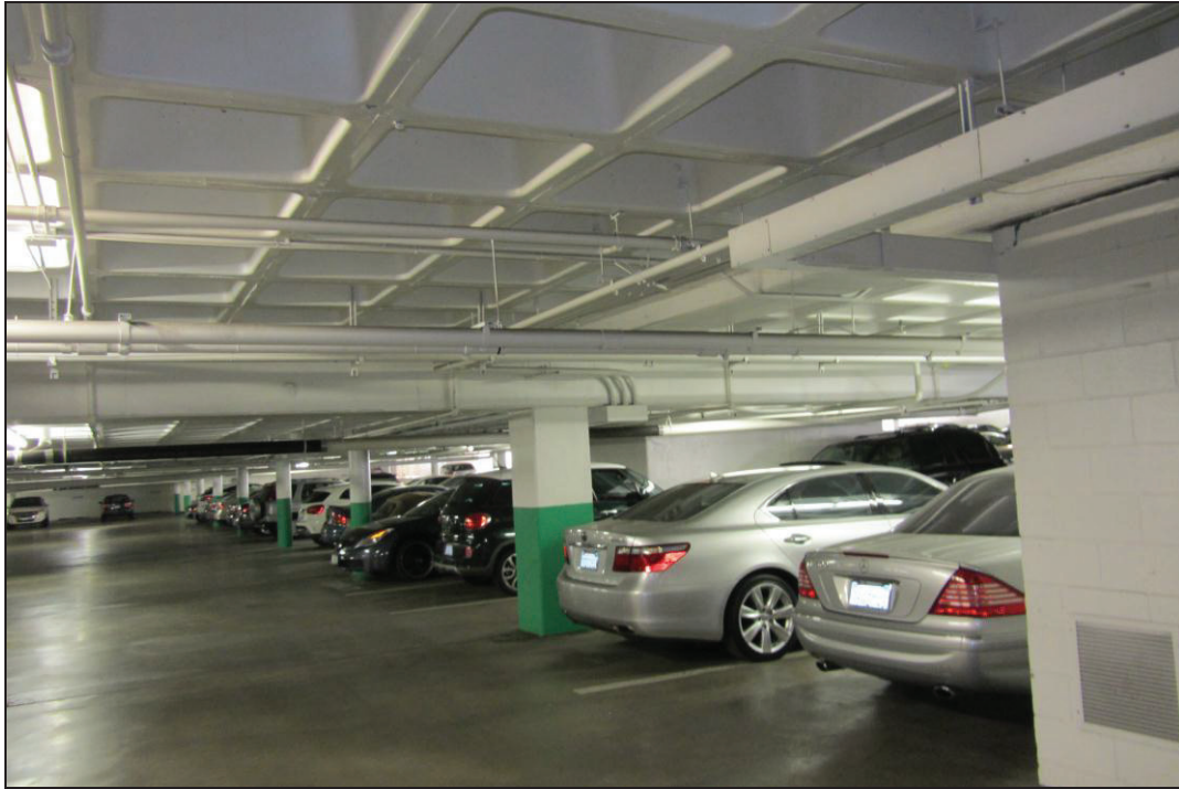
Photo 3 – Typical First Floor Framing
