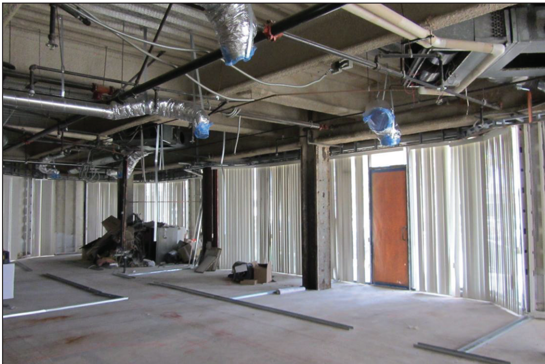
Photo 4 – Typical Steel Framing
