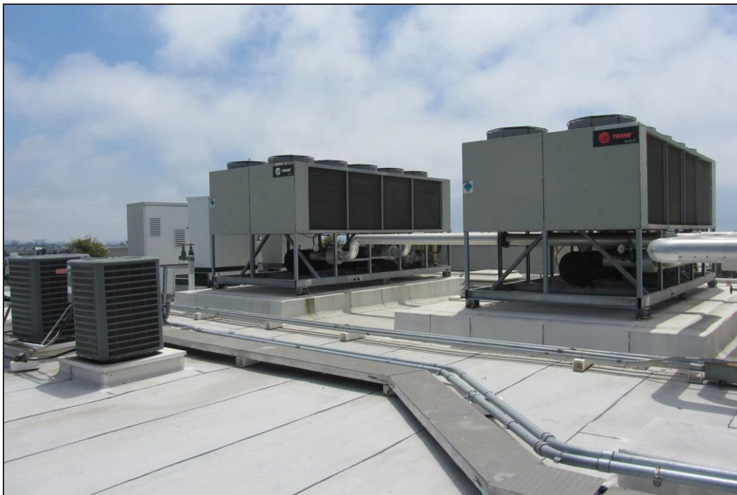
Photo 6 – Rooftop Cooling Towers
