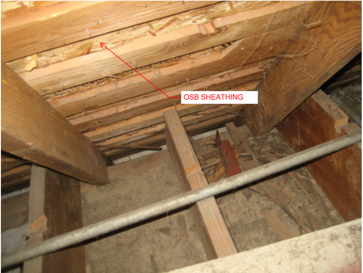
Figure 2.3 As-built Roof Diaphragm Picture
