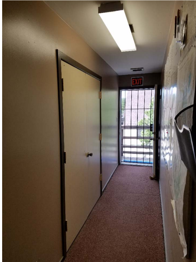
Figure 8: Main Building Corridor
