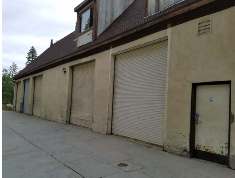
Figure 6: Main Building (Rear)
