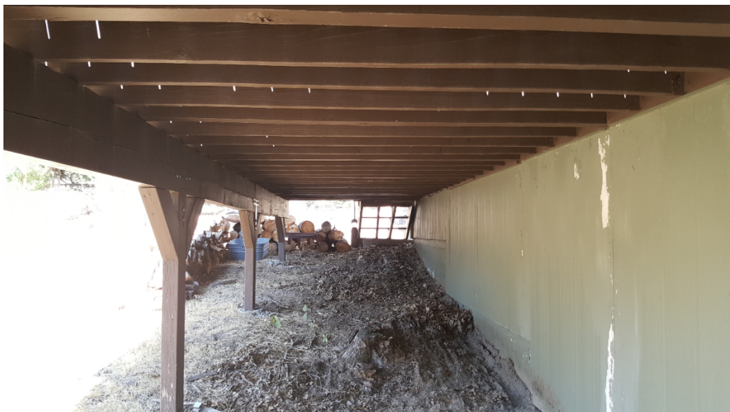
Figure 5: Underside of Rear Balcony / Deck
