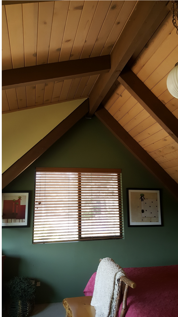
Figure 7: Roof Framing / Ridge Beam
