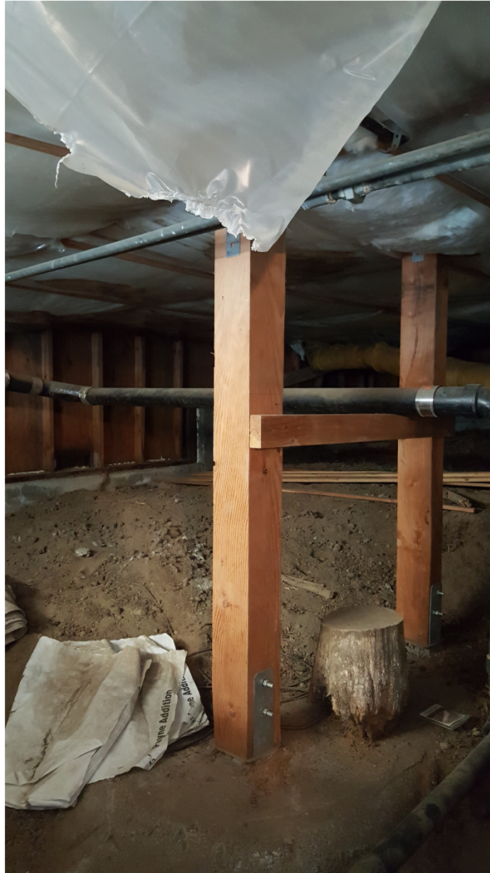
Figure 9: Basement Cripple Walls
