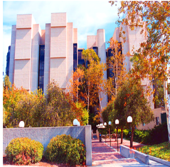
9) Exterior Elevation Photo
