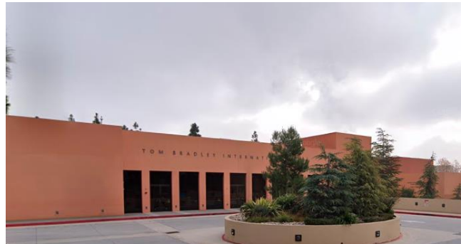
Exterior Elevation Photo
