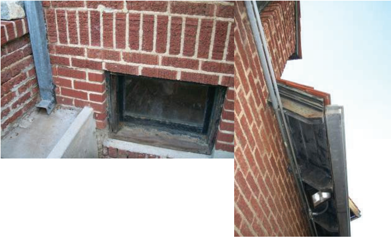
Photo B.1: Exterior Rafter Tail and Window Frame Deterioration
