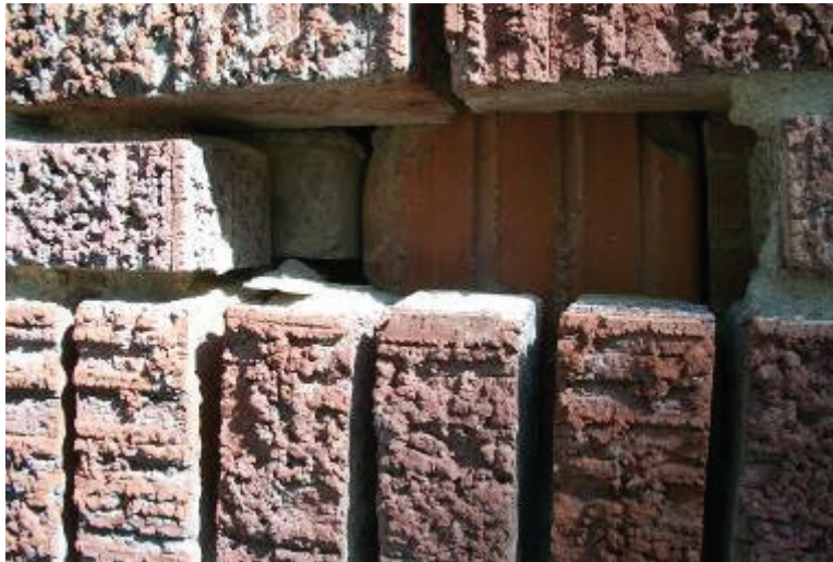
Photo B.6: Exposed HCT at Exterior
