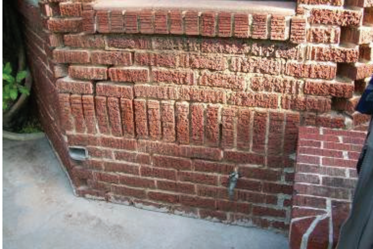
Photo B.3: Mortar Deterioration at Façade Brick
