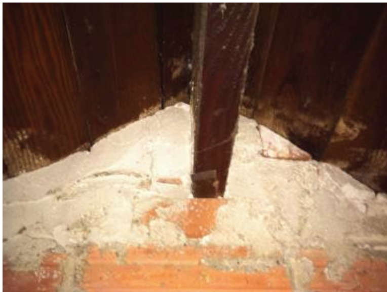
Photo B.5: Roof Framing to Exterior HCT Walls
