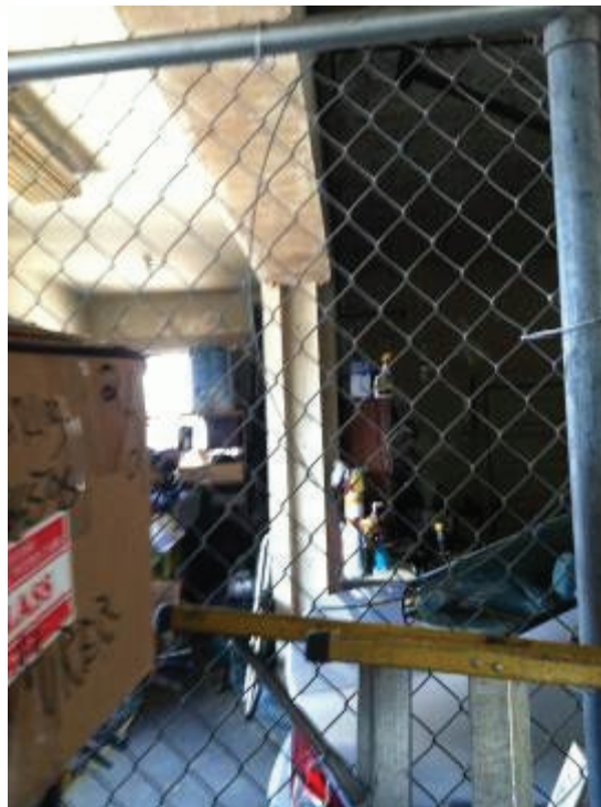
Photo B.7: Steel Column and Beam at Opening
