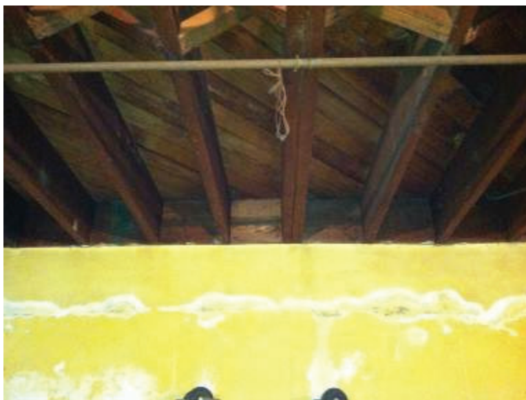
Photo B.4: Basement Wall Crack
