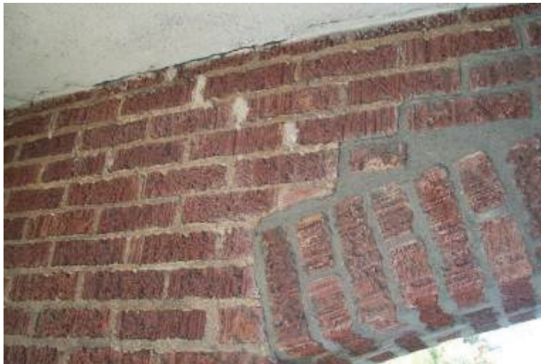
Photo B.2: Repointed Mortar and Plaster Cracks
