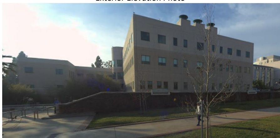
Exterior Elevation Photo
