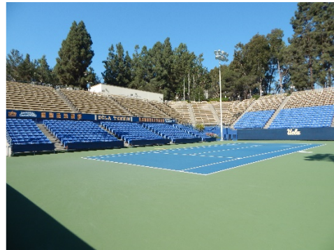
Exterior Elevation Photo
