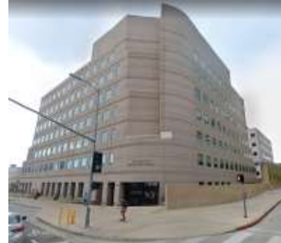
Exterior Elevation Photo
