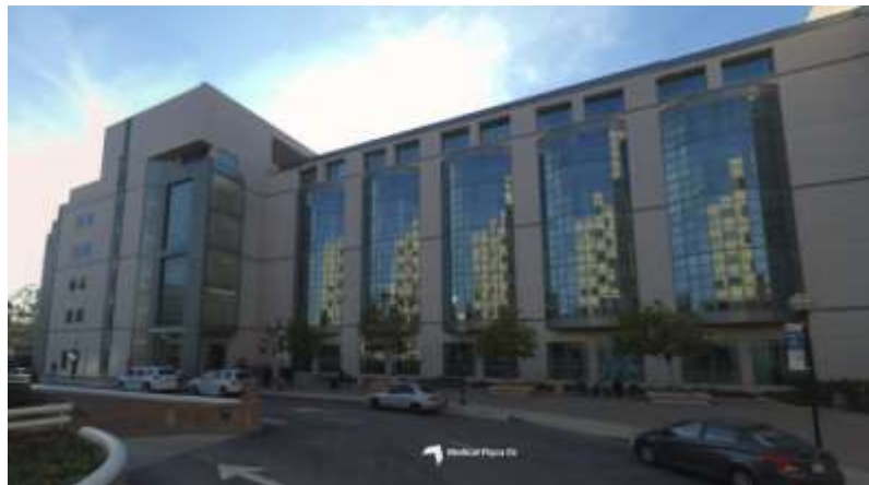
Exterior Elevation Photo
