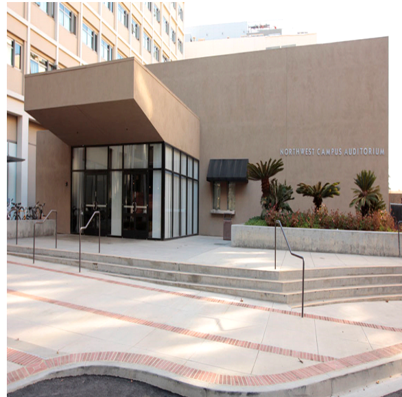
9) Exterior Elevation Photo
