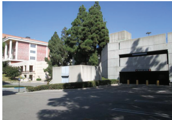
West Elevation of the Parking Structure
