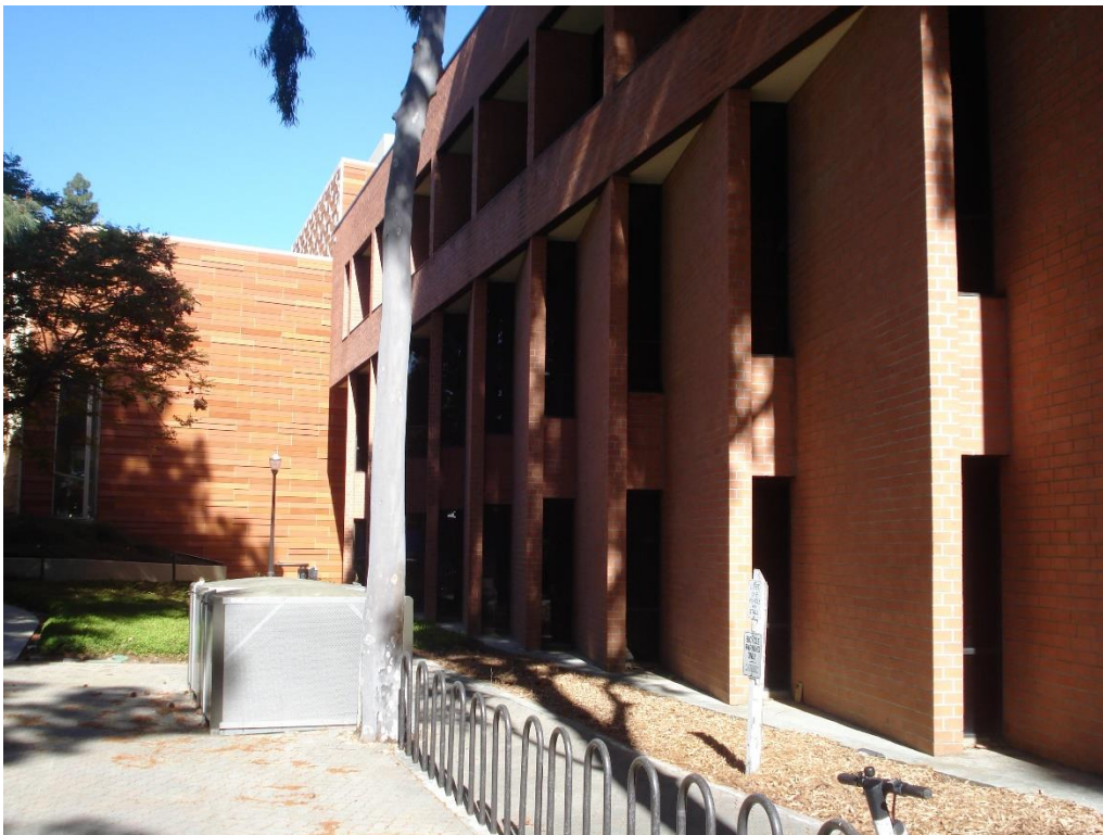
South side of Building – Discontinuous 2 nd floor pier straddling skewed walls from ground to 2 nd floor.
