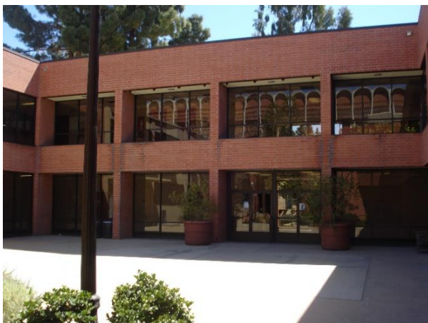
Westside of Building - Courtyard Elevation at first floor
