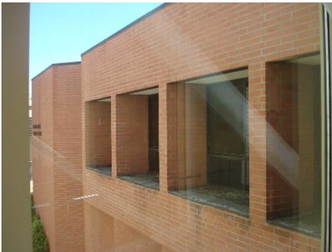
West side of building - Brick piers at 2 nd floor
