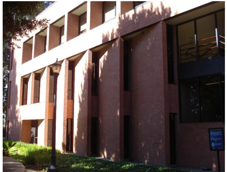
Exterior Elevation Photo – East Side of Building
