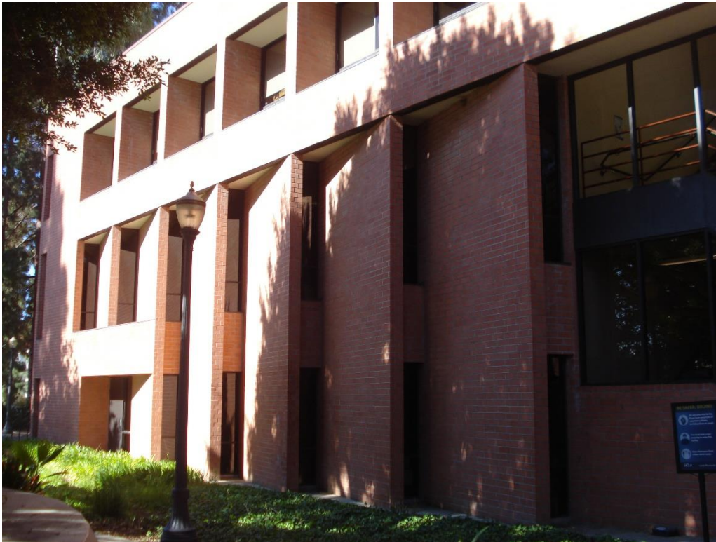
East side of building – Discontinuous piers, skewed walls and skewed wall sits on lintel.
