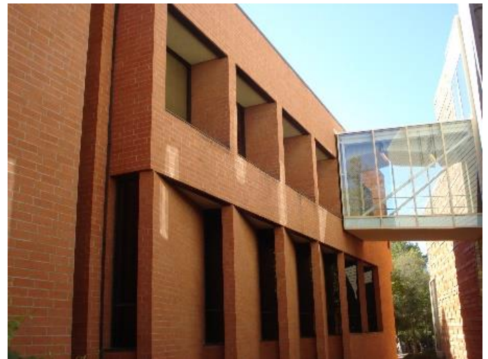
West side of building: Brick piers at 2 nd floor, skewed walls at first floor
