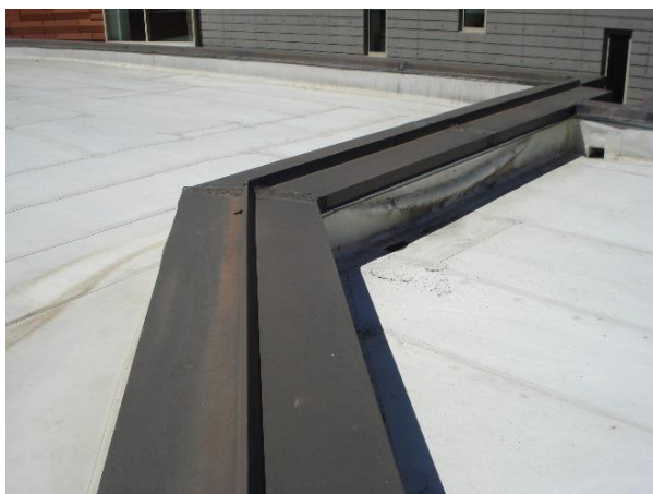
Seismic joint / flashing at Organ Chamber Building With Herb Albert Building
