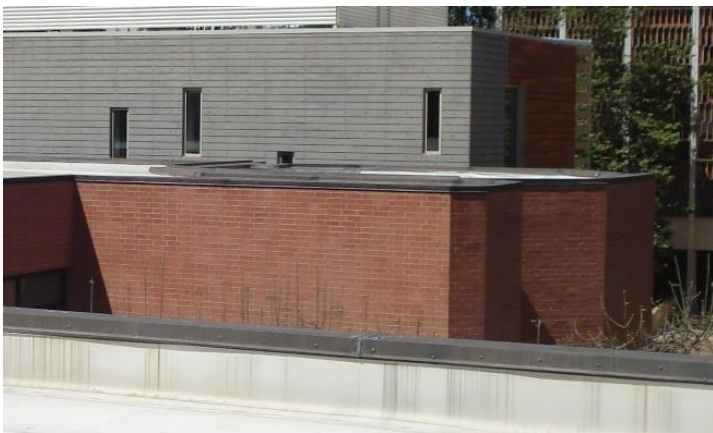
Organ Chamber & Stairwell – looking west
