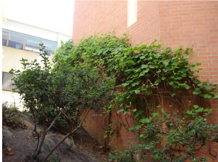
Exposed west wall (ground floor to first floor) showing brick veneer over concrete wall.
