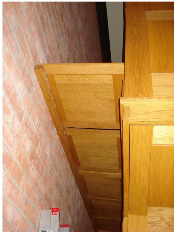
Existing organ wall bracing
