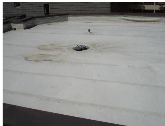
Seismic joint cover and top of wall flashing
