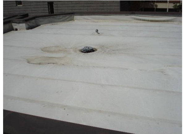
Organ Chamber Roof - some loose roofing at parapet
