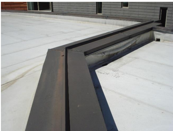
Seismic joint cover / flashing at roof south edge
