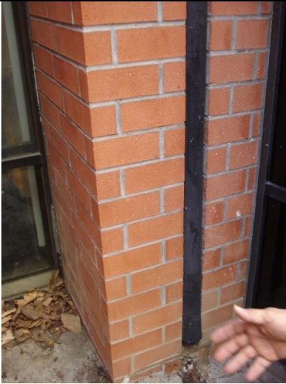
Seismic joint in wall at ground floor level (West side of building) in need of review and/or replacement cover.
