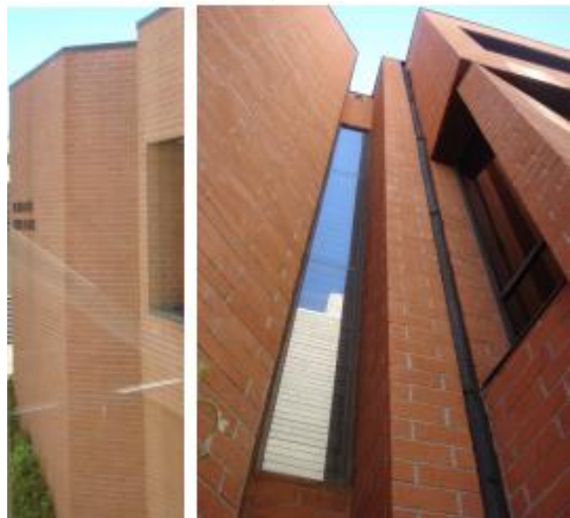
Left: West Elevation, Right: Seismic Joint
