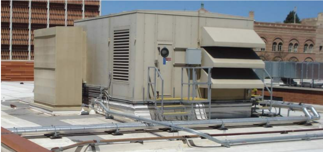
Mechanical Unit #1 (south end of building)
