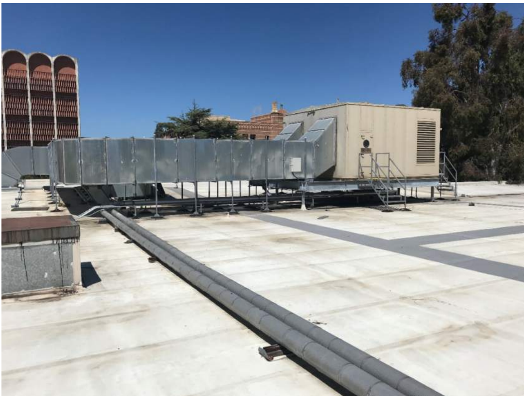
Mechanical Unit #2 (north end of building)
