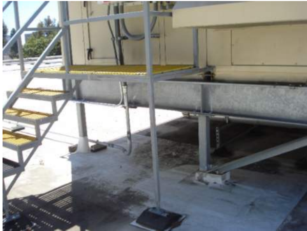
Mechanical Unit #2 supports
