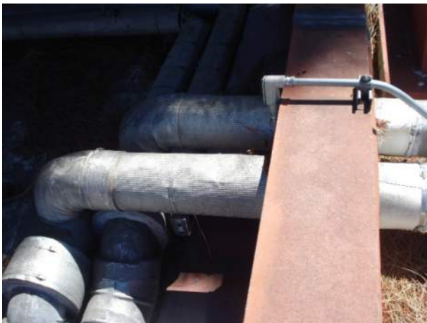
Water pipes and conduit crossing seismic joint with no visible flexible connections provided.
