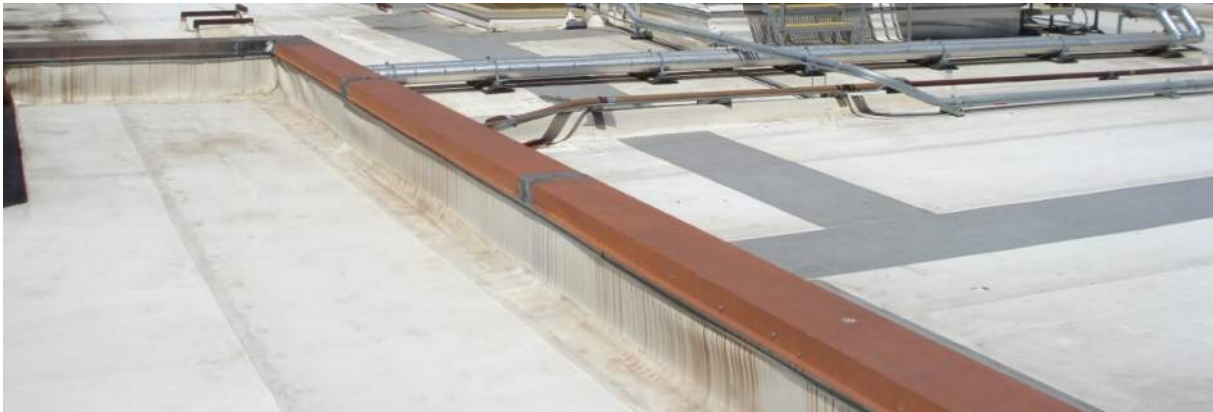
Parapet wall flashing cover that serves as seismic joint cover where two adjacent buildings occur
