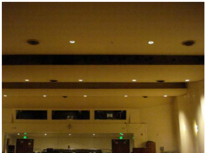
Main auditorium ceiling – three ceiling sections
