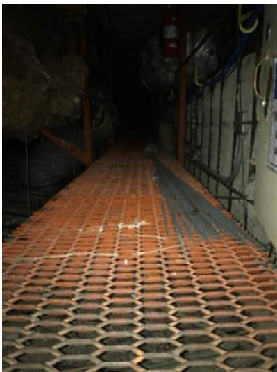
Catwalk framing above main auditorium (catwalk shown in ceiling section above)
