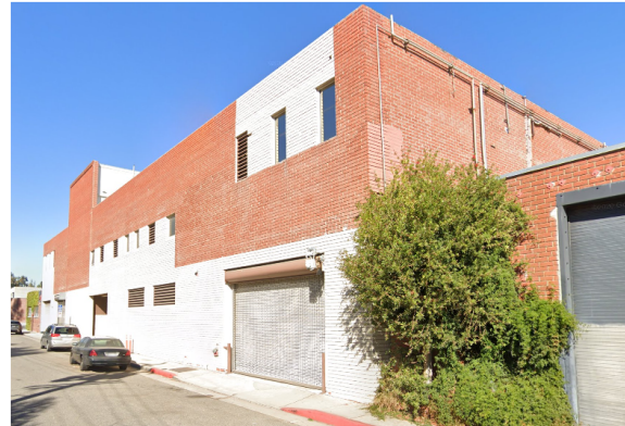
Exterior Elevation Photo
