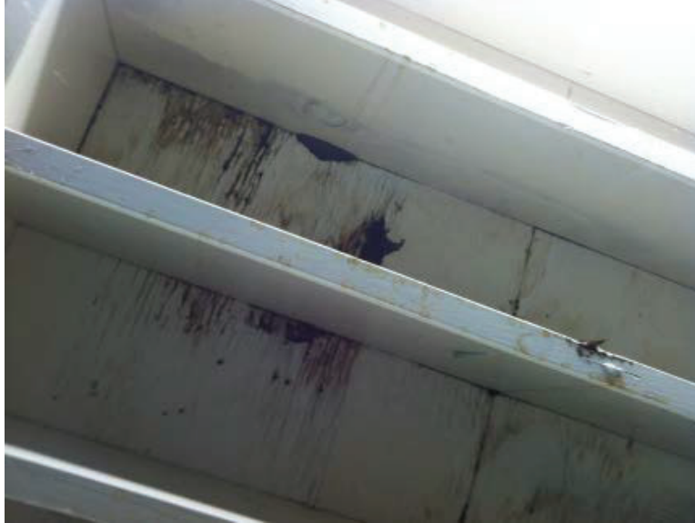
Photo 3.6: Building P: Roof Sheathing Damage
