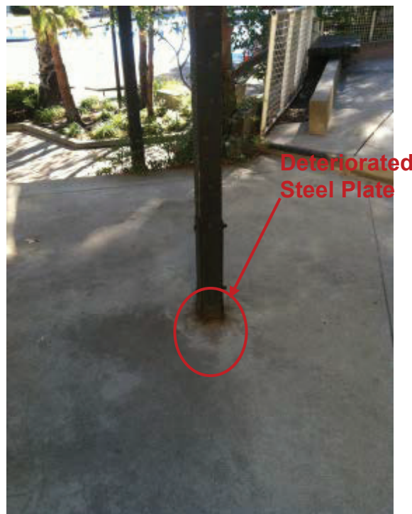
Photo 3.5: Trellis Post to Slab Connection
