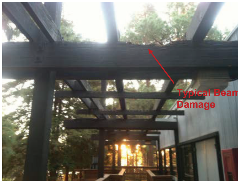
Photo 3.1: Exterior Walkway at Building B – Beam Damage
