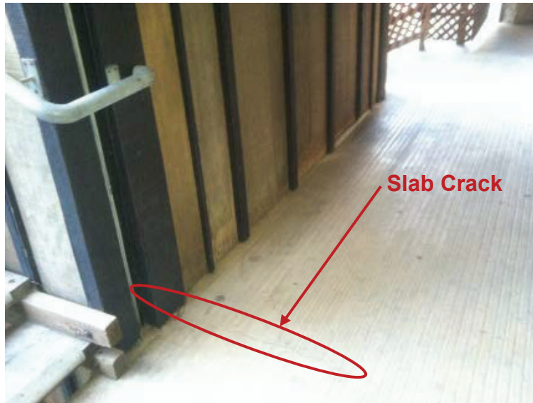
Photo 3.4: Building D/F: Concrete Slab Cracks at Connection
