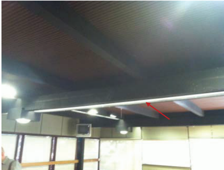
Photo 3.2 : Interior Building C - Deflected Roof Beam
