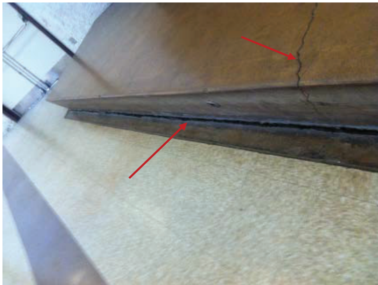
Photo 3.3: Interior Building D - Concrete Cracks at Stage
