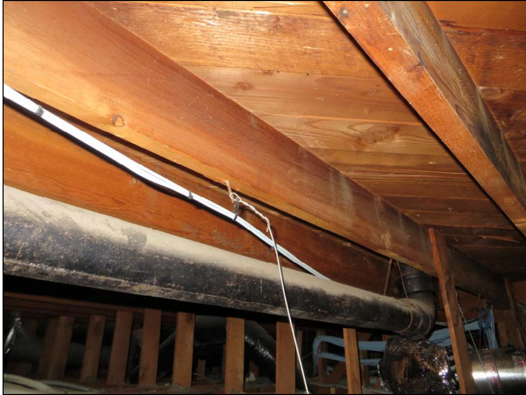
Photo 4 – Typical Wood Framing
