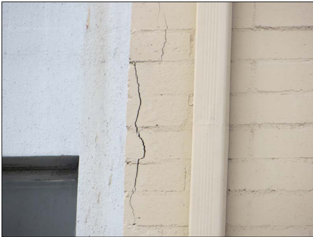
Photo 4 – Crack in Masonry Wall at Northwest Corner
