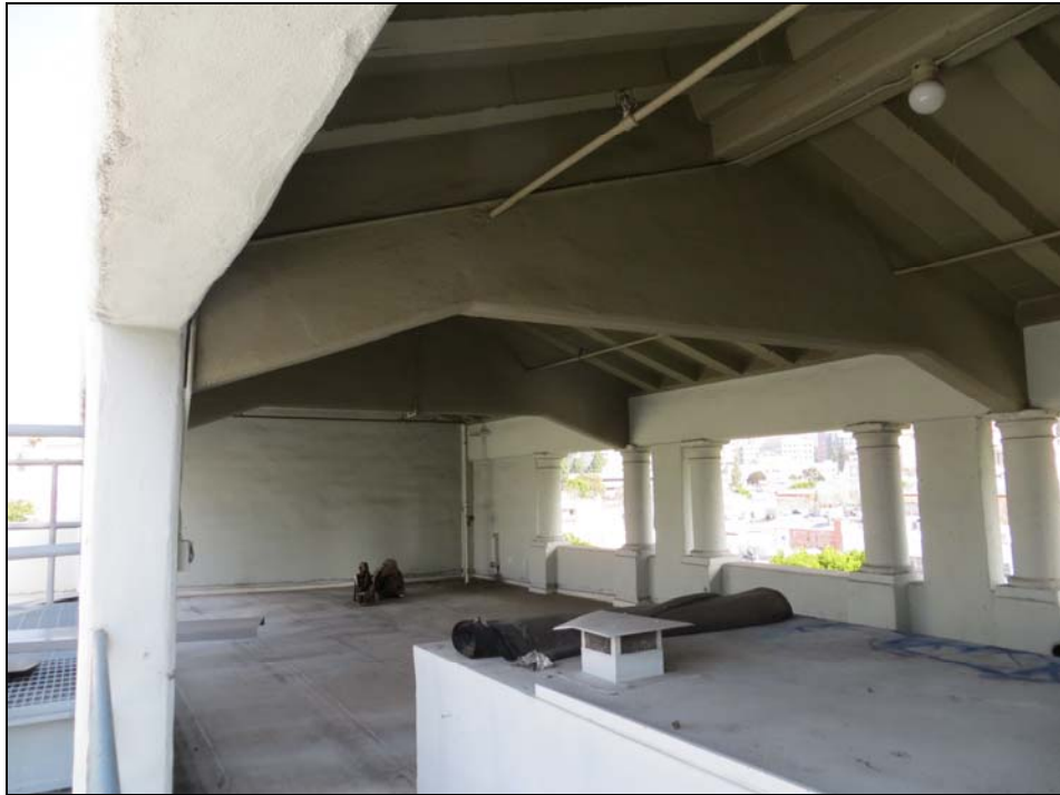
Photo 5 – Typical Concrete Framing at Penthouse
