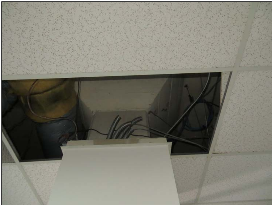
Photo 4 – Typical Column Capital
