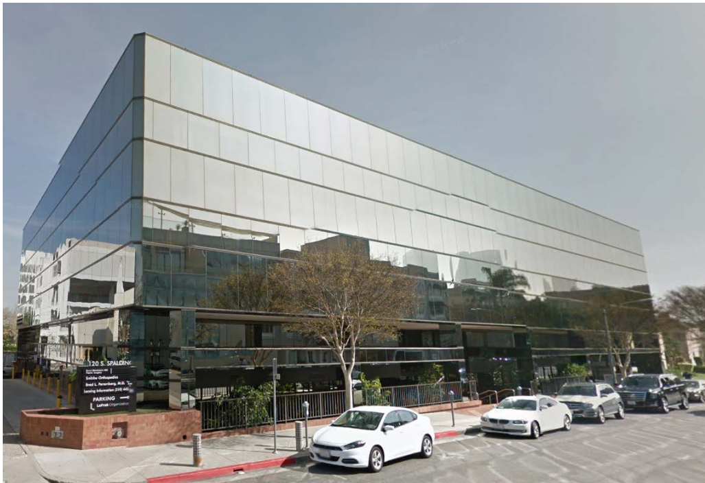
South elevation of 120 Spalding Ave, Beverly Hills, CA.
