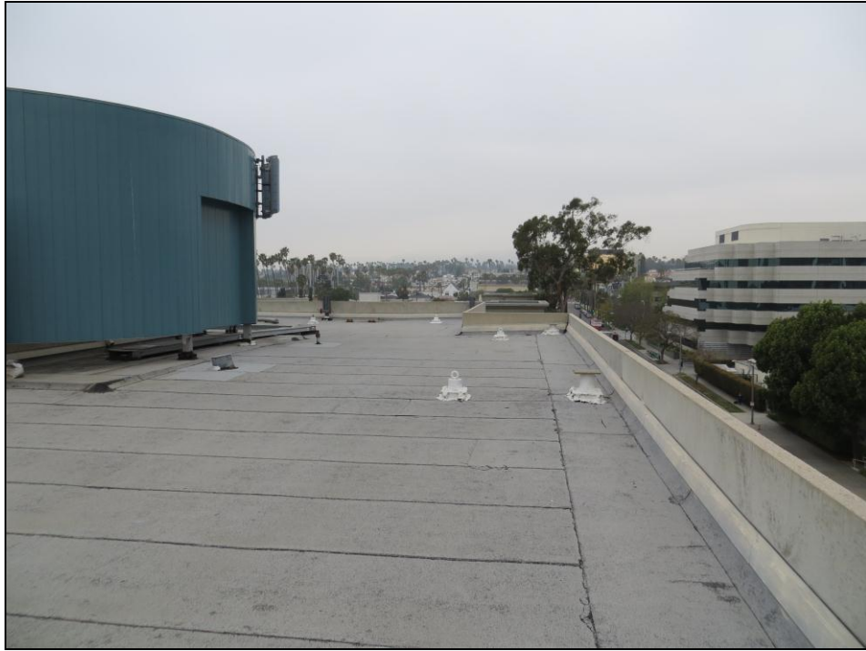
Photo 9 – Main Roof and Parapet
