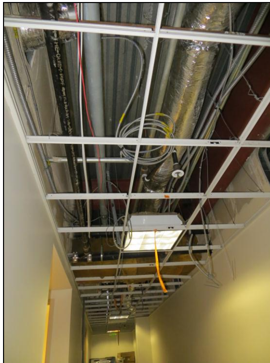
Photo 10 – Typical Piping and Ductwork
