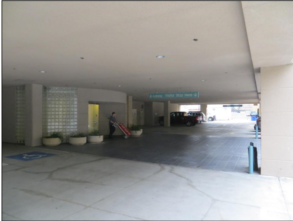
Photo 7 – Driveway (1 st Floor)
