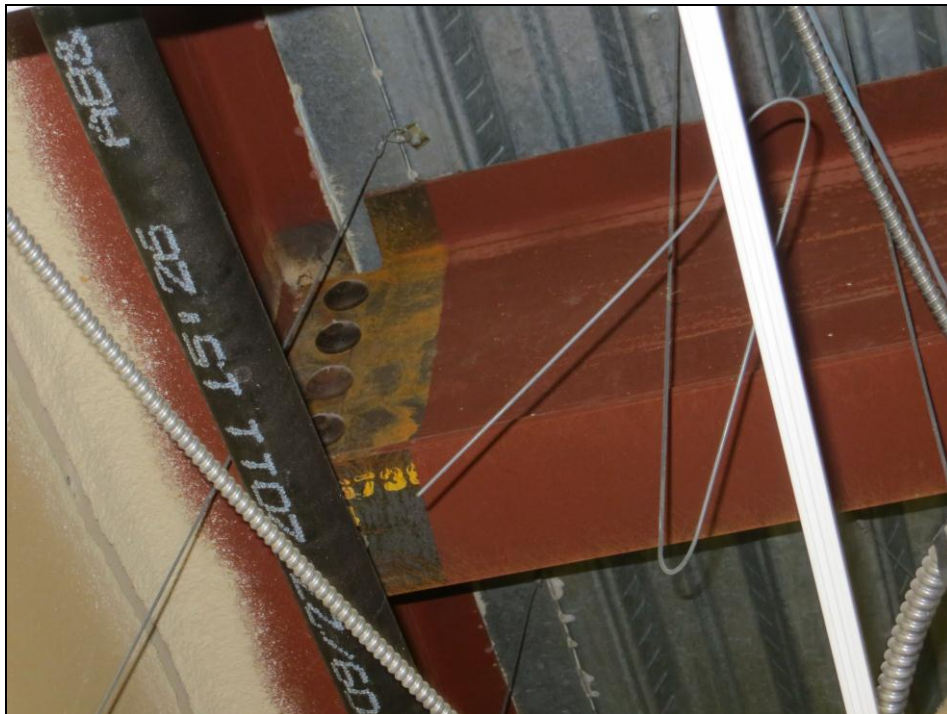
Photo 8 – Typical Steel Framing
