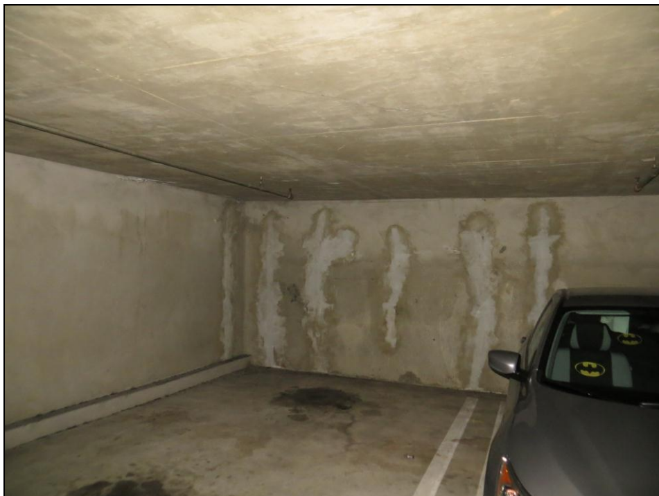
Photo 6 – Concrete Retaining Wall
