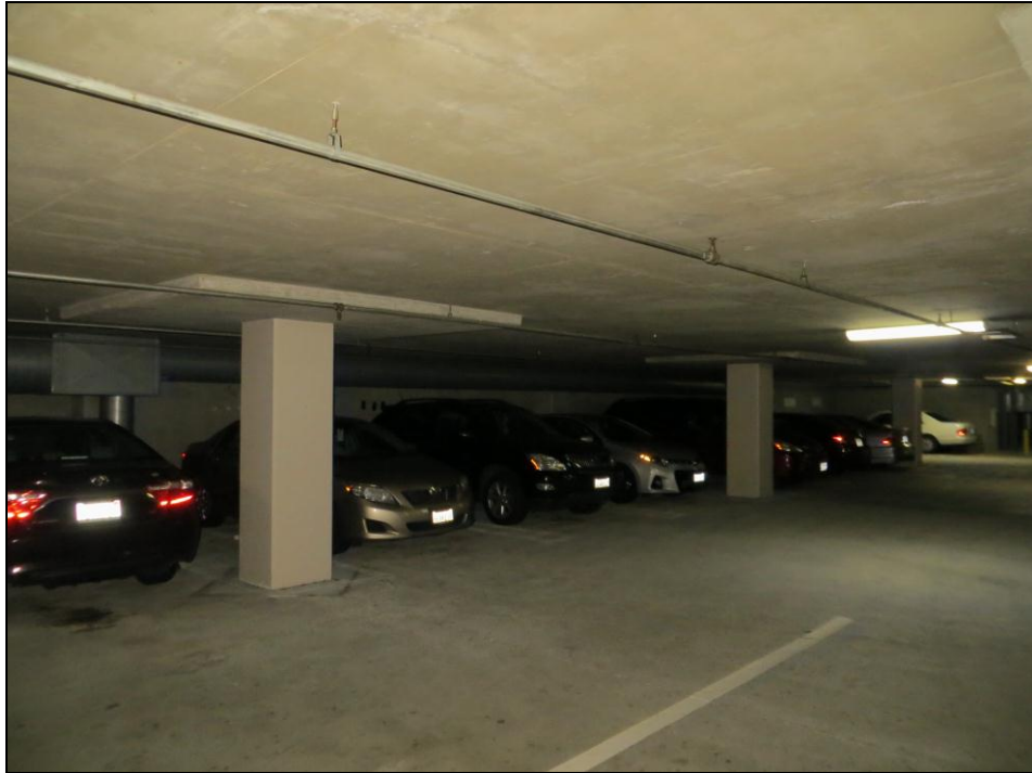
Photo 5 – Typical Concrete Framing Subterranean Parking
