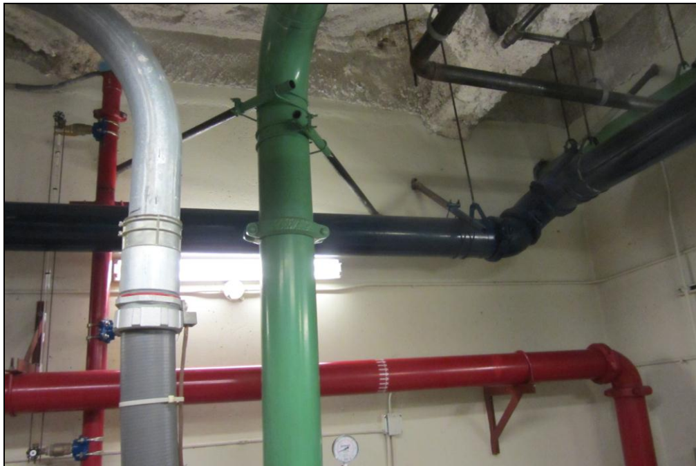
Photo 8 – Bracing of Piping Systems
