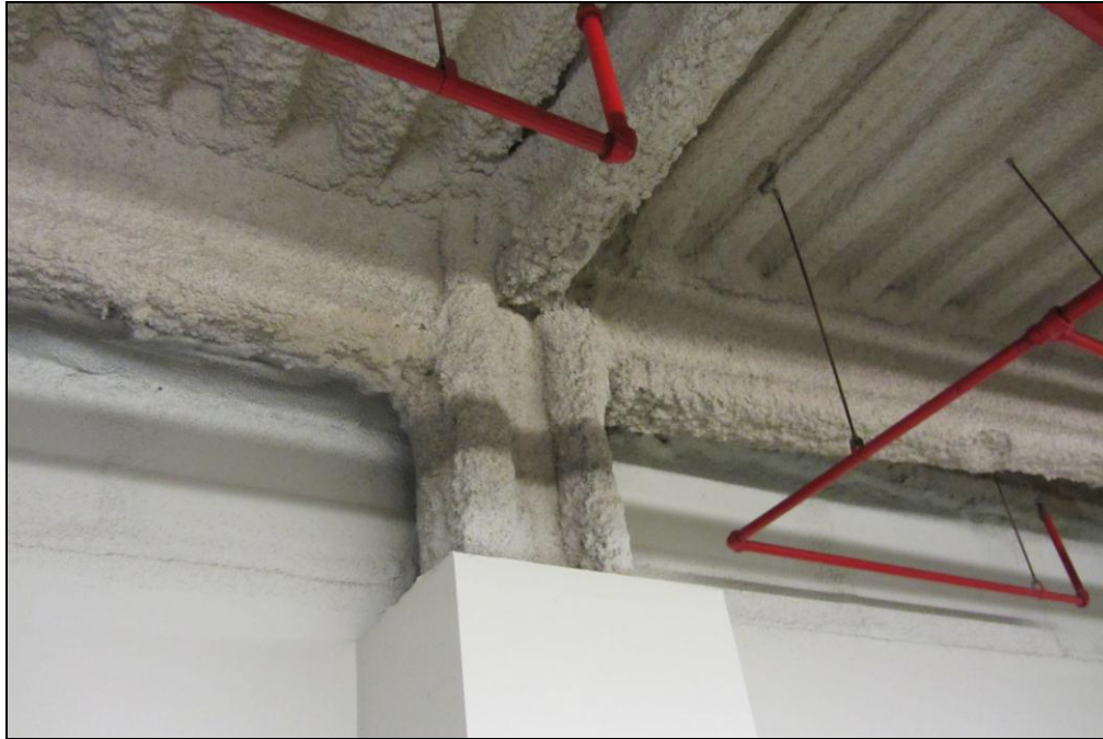
Photo 5 – Typical Beam to Column Connection
