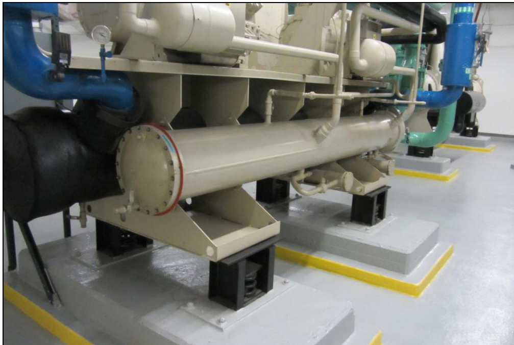
Photo 6 – Anchorage of Mechanical Equipment
