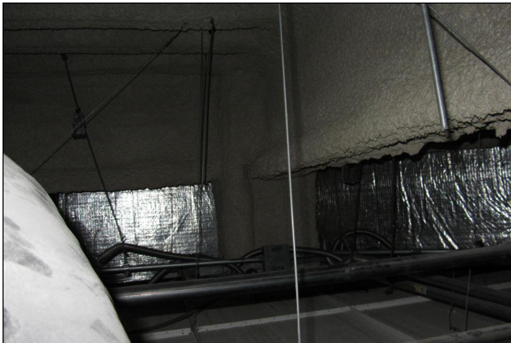
Photo 4 – Typical Beam to Column Connection
