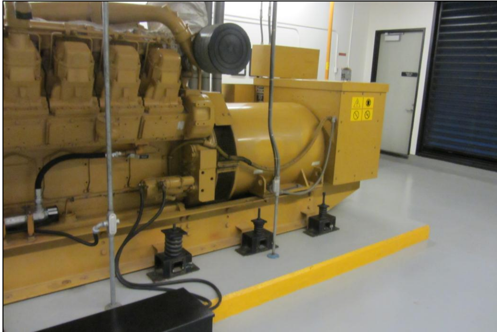
Photo 7 – Anchorage of Emergency Generator
