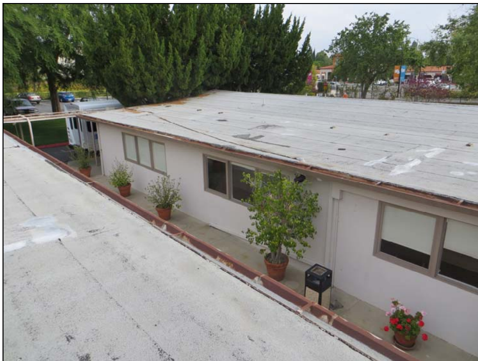
Photo 2 – West Elevation of East Wing
