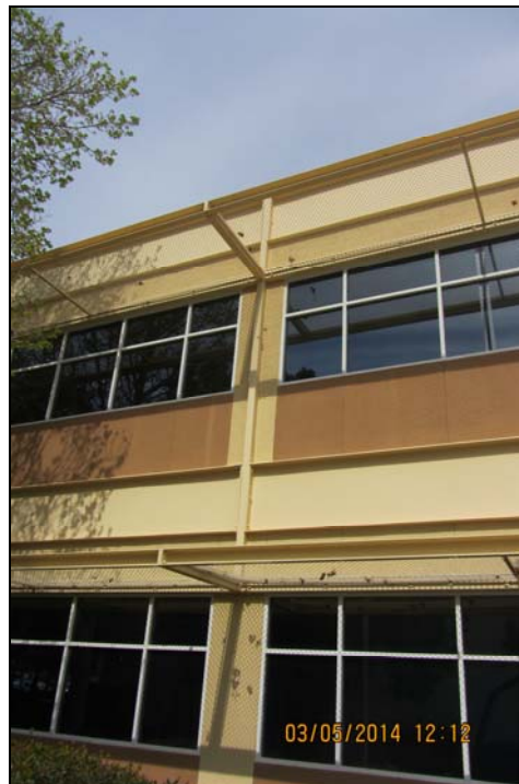
Photo 4 – Steel Framed Screen Awning
