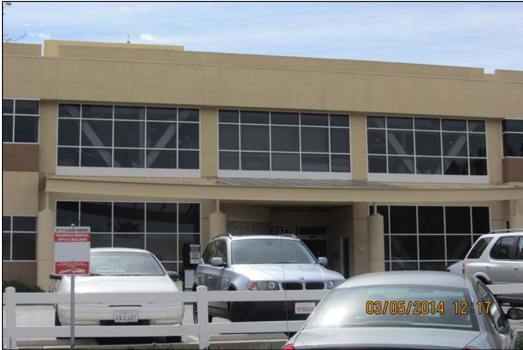
Photo 3 – Steel Braced Frames
