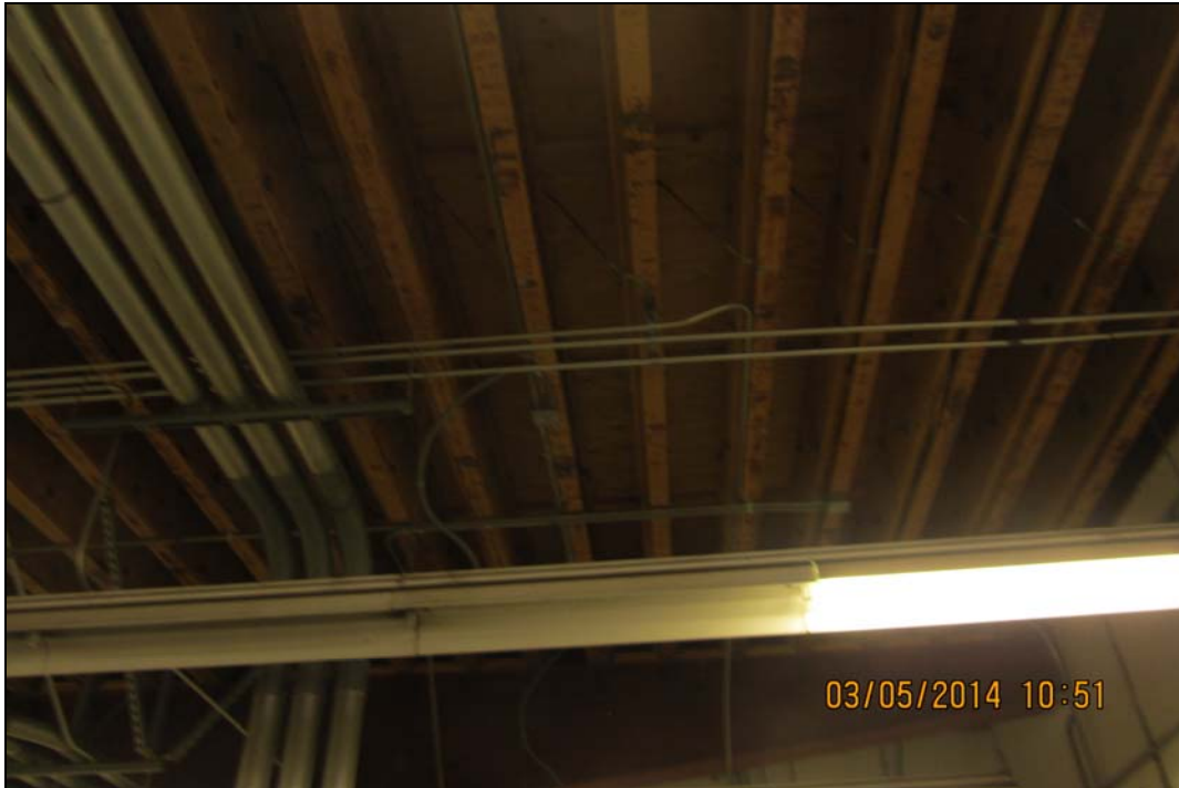
Photo 3 – Typical Floor Framing
