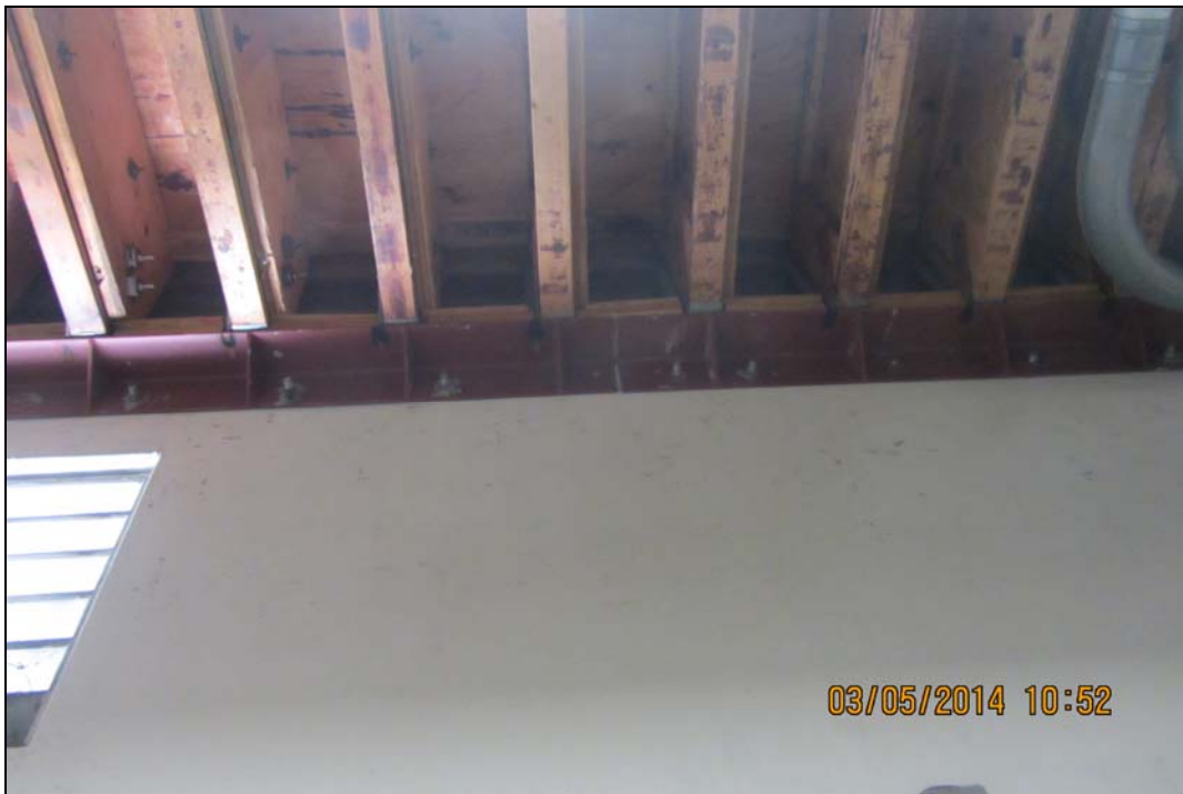
Photo 4 – Typical Joist to Wall Connection
