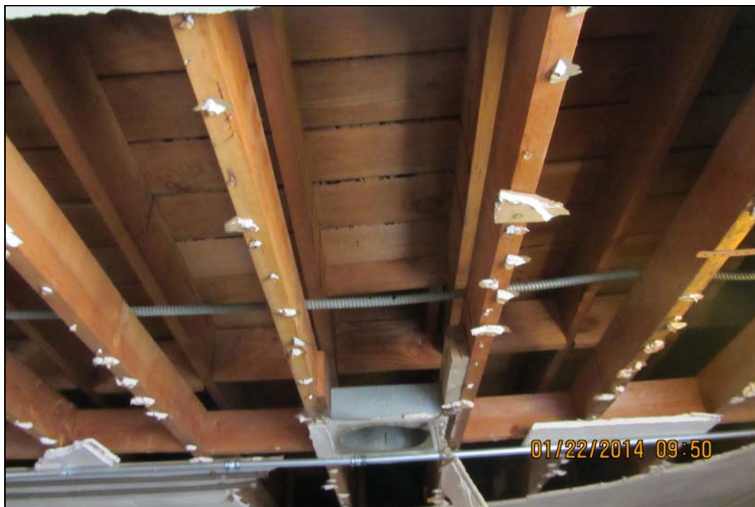
Photo 4 – Wood Framed Roof
