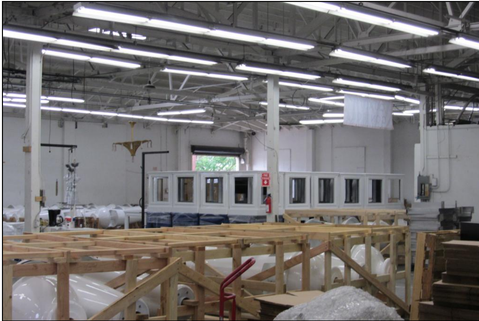
Photo 5 – Wood Posts and Roof Framing
