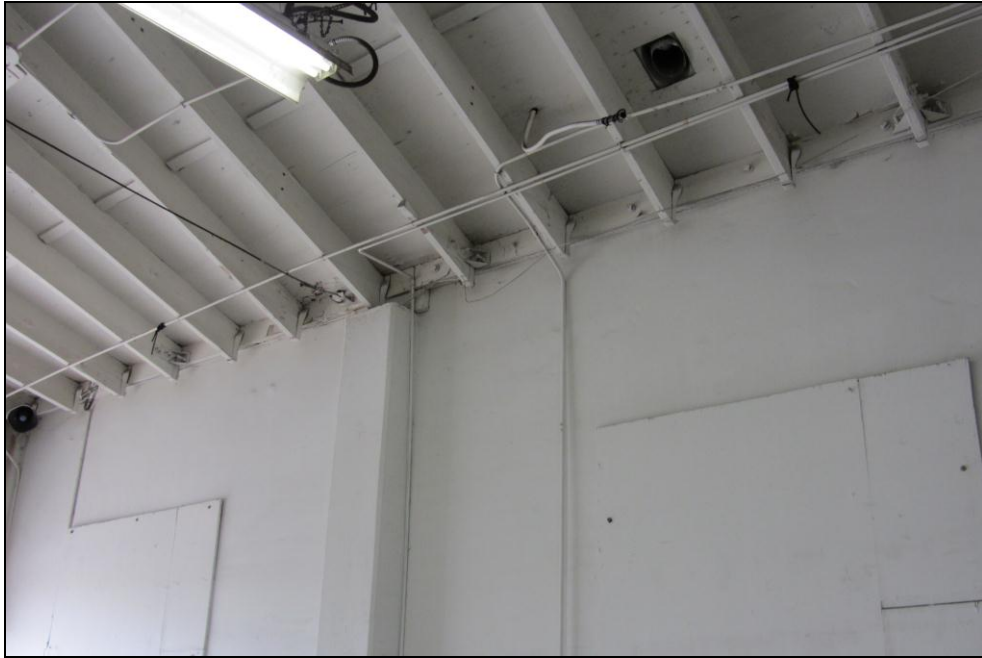
Photo 7 – Out-of-Plane Wall Anchors at Rafters
