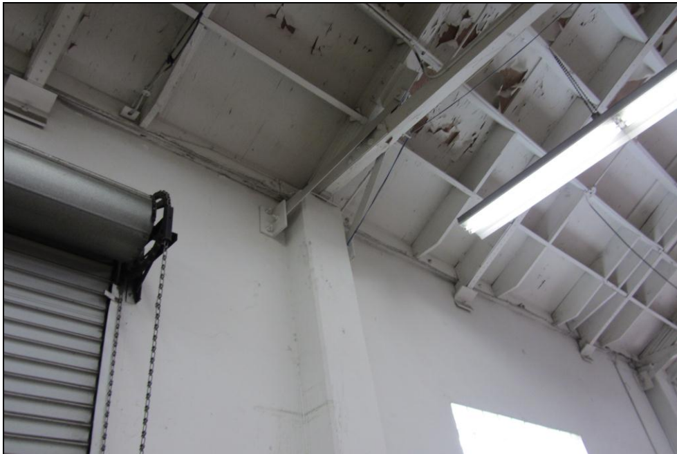
Photo 6 – Out-of-Plane Wall Anchors at Pilaster
