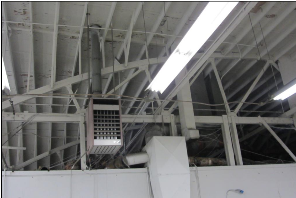
Photo 8 – Unbraced Hanging AC Unit
