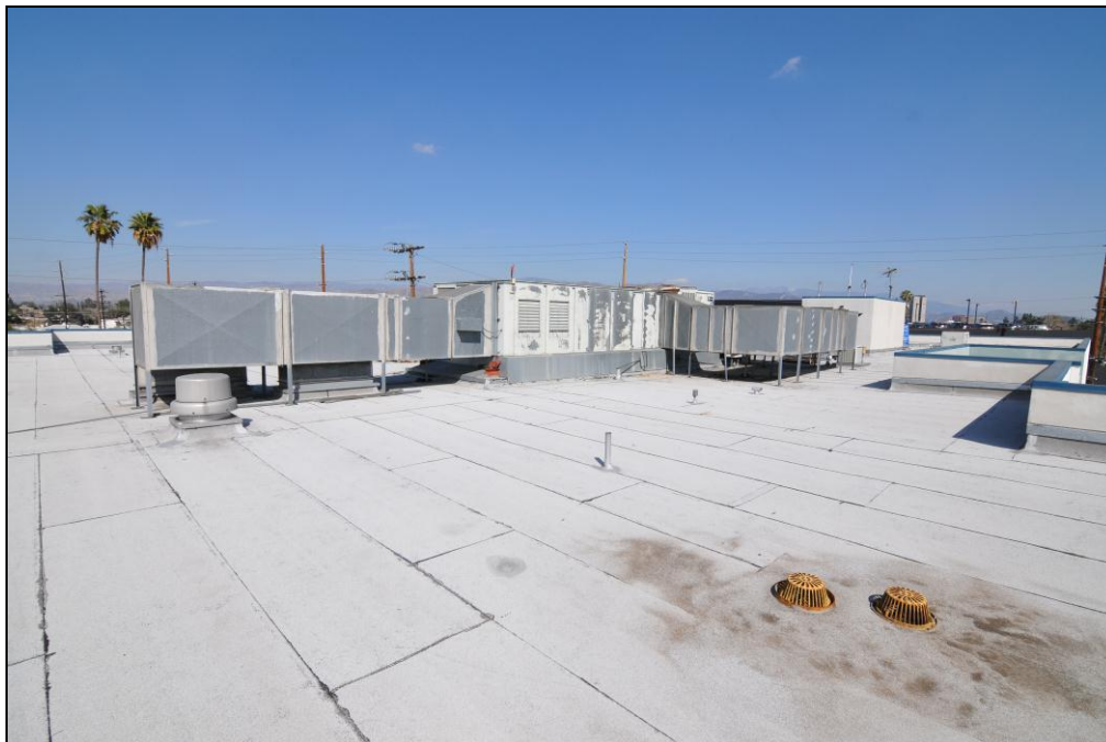
Photo 8 – HVAC Units on Roof
