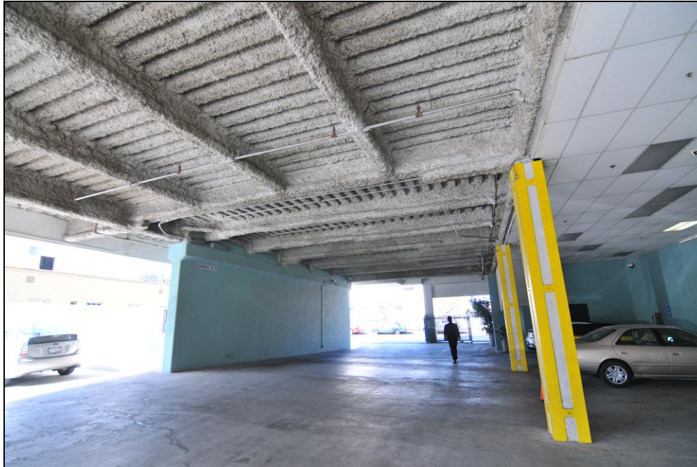
Photo 7 – Typical Steel Framing and Concrete Shear Wall
