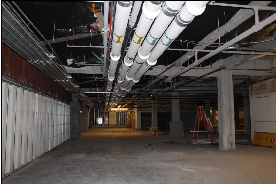
Photo 3 – Braced Piping
