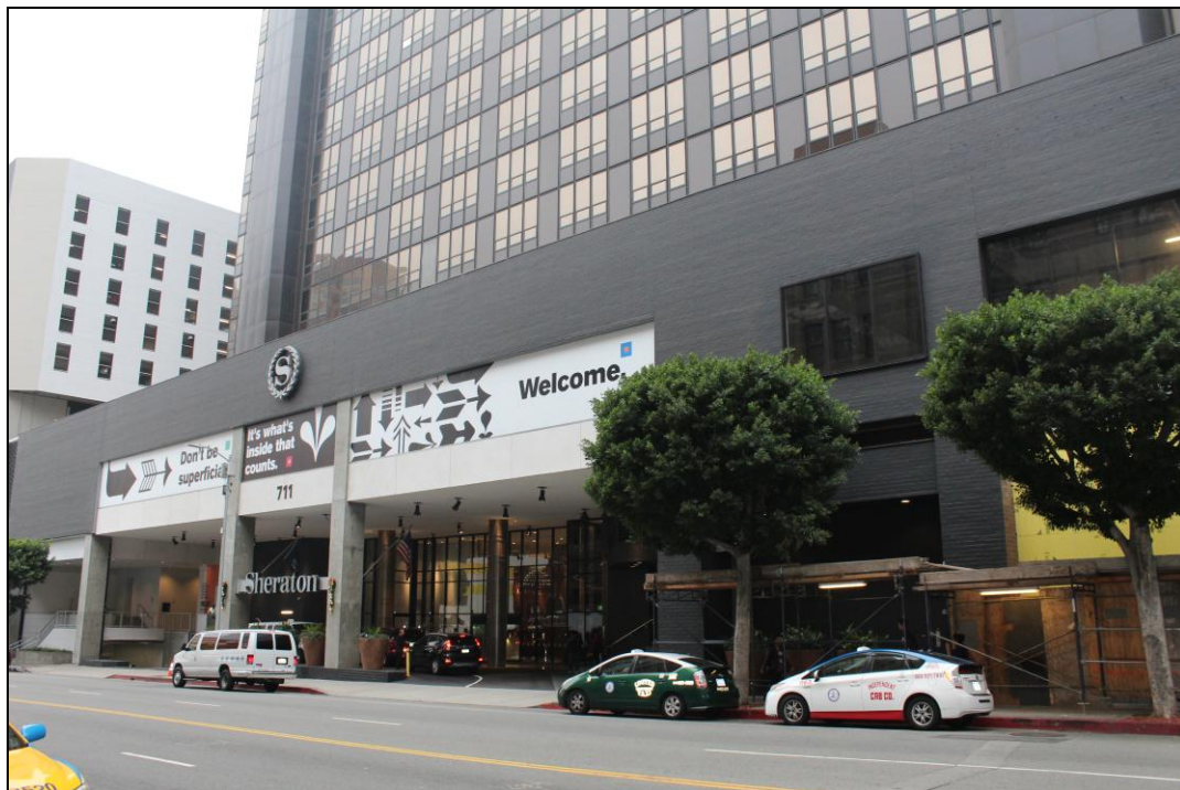
Photo 2 – East Elevation (Low-Rise)
