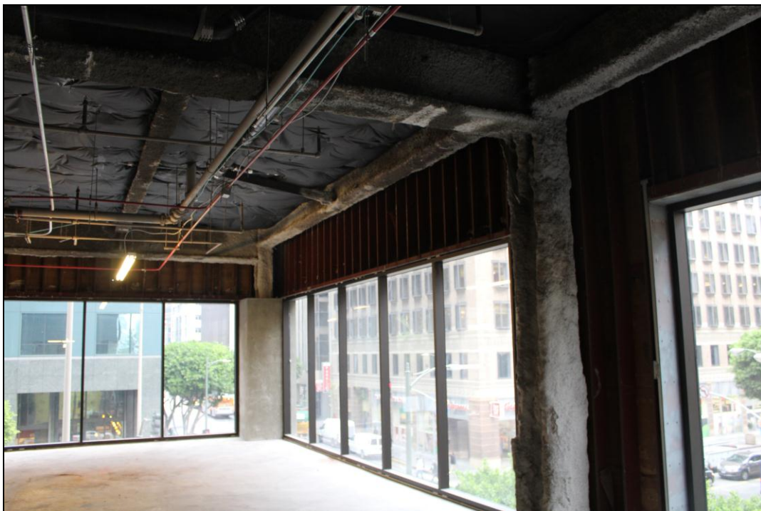
Photo 4 – Typical Steel Framing
