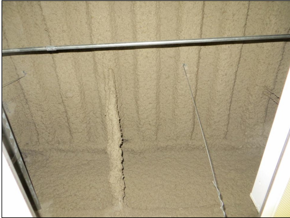
Photo 3 – Metal Deck and Steel Framing
