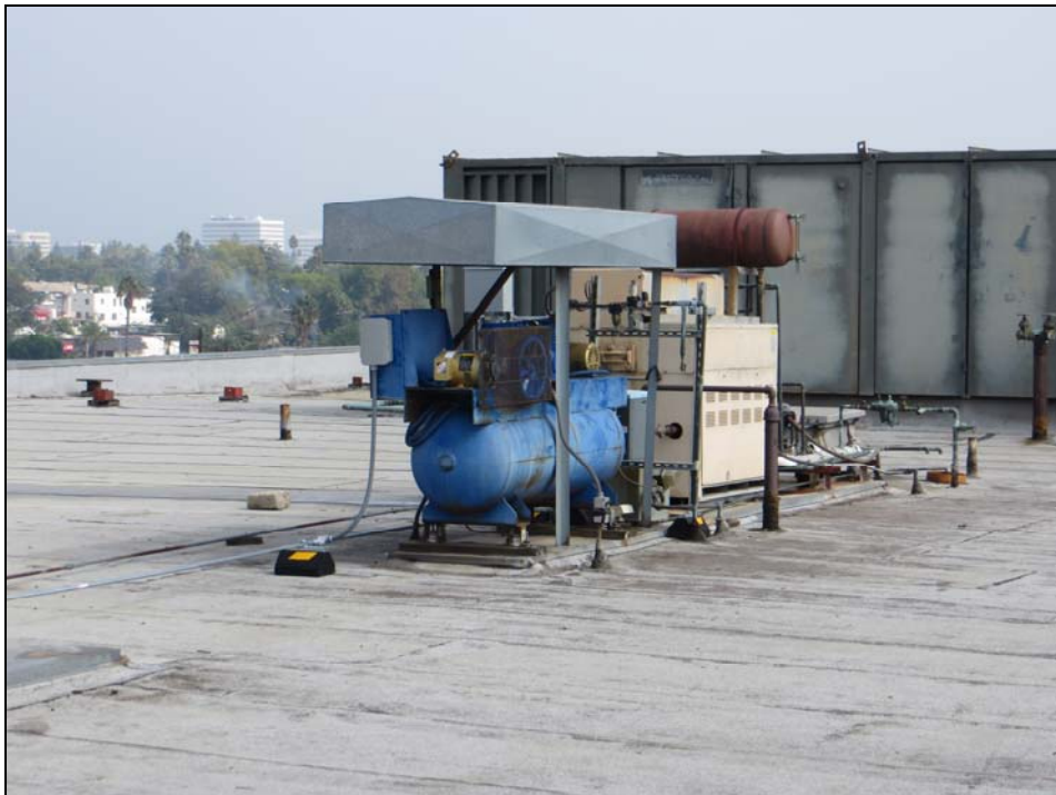
Photo 4 – Mechanical Equipment on Roof
