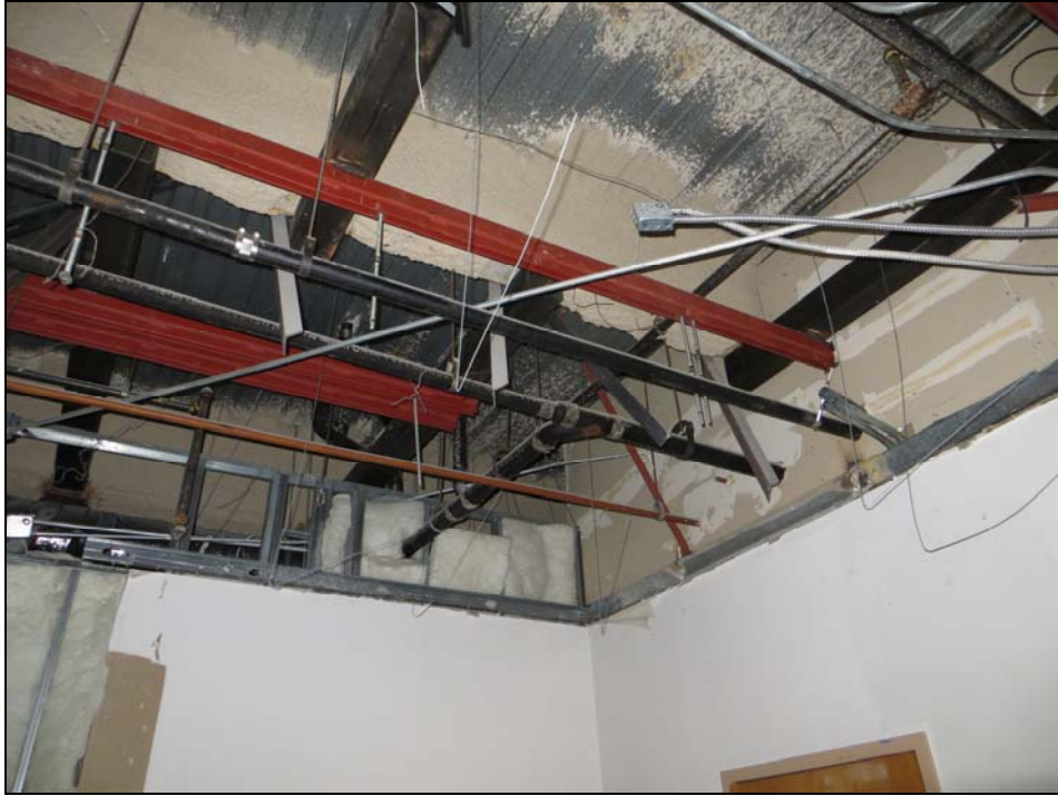
Photo 3 – Steel Framing with Braced Partition and Piping
