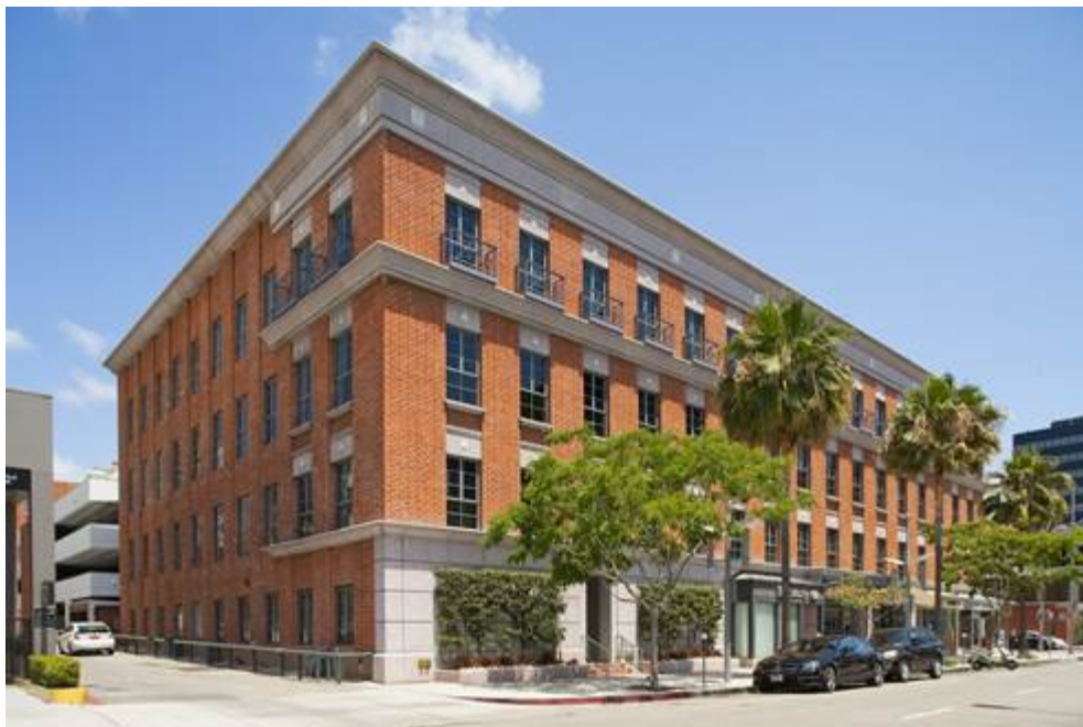
Southwest elevation, 9675 Brighton Way, Beverly Hills, CA
