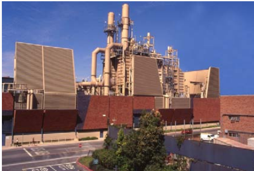
Facilities Management Building (Cogeneration Plant)
