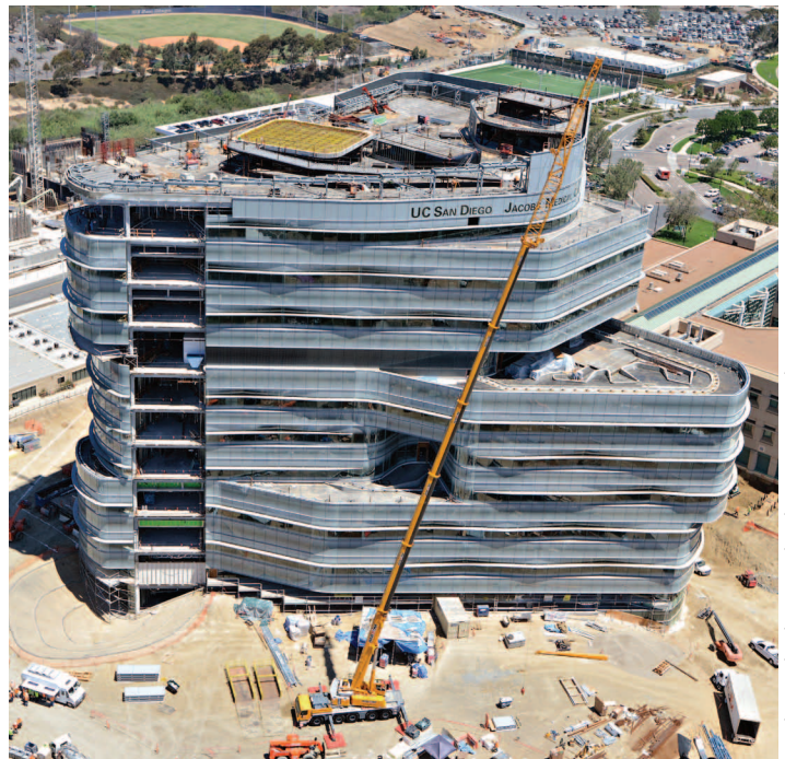
Jacobs Medical Center (under construction)
