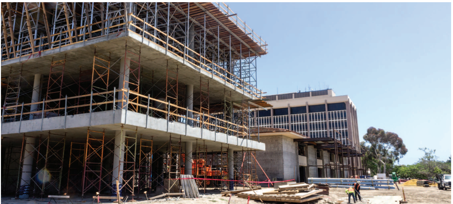
Davidson Library Addition and Renewal (Under Construction)
