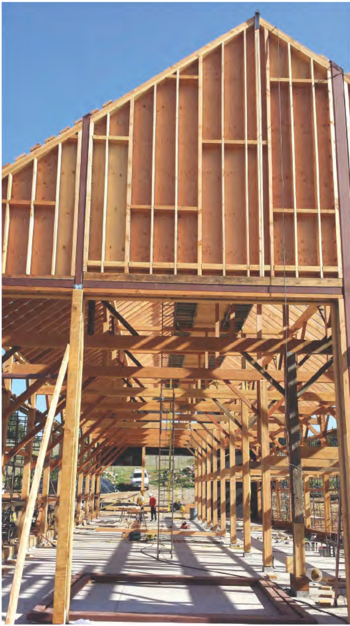
Barn (In Construction)
