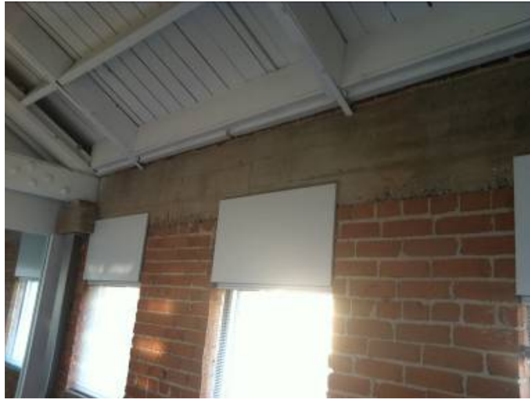
Photo 3: URM Wall to Roof Framing Connections
