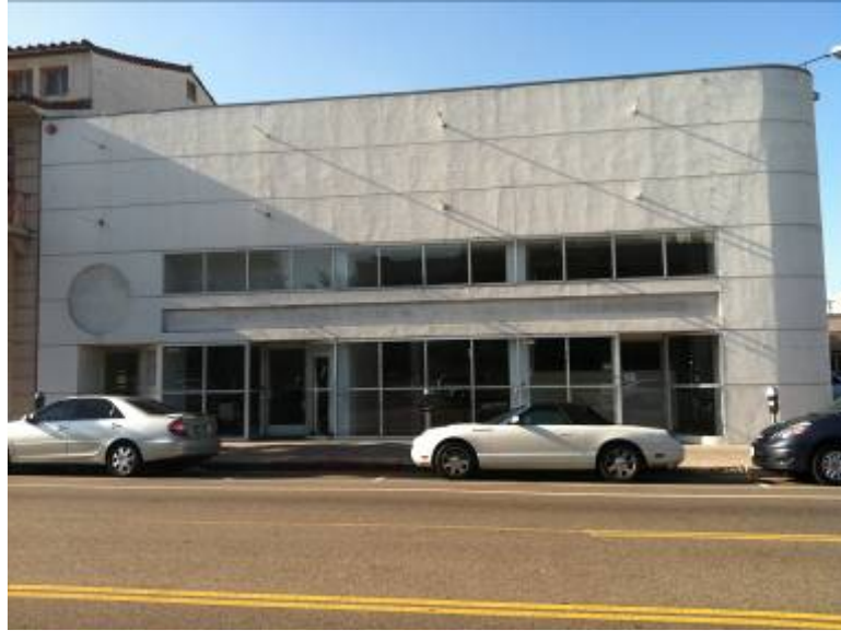
Photo 1: Exterior View of Building – North Facing Wall
