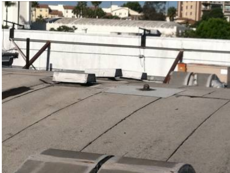
Photo 4: Parapet Wall Bracing
