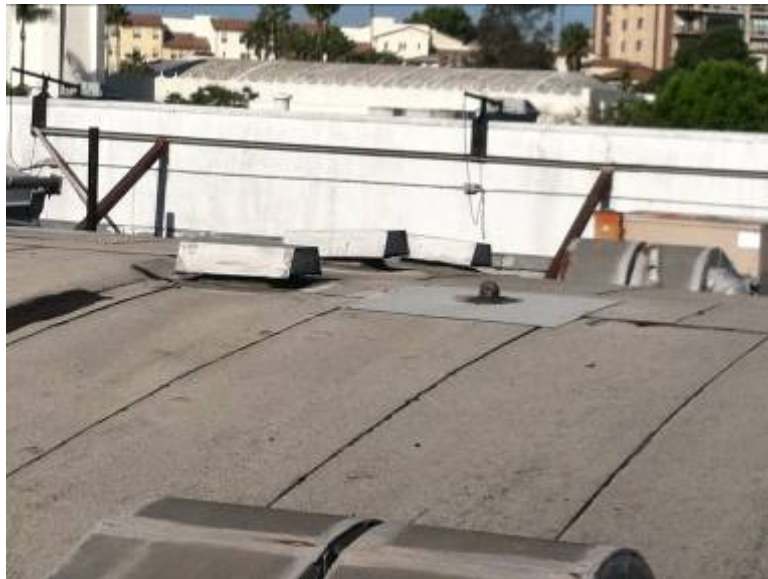
Photo 4: Parapet Wall Bracing
