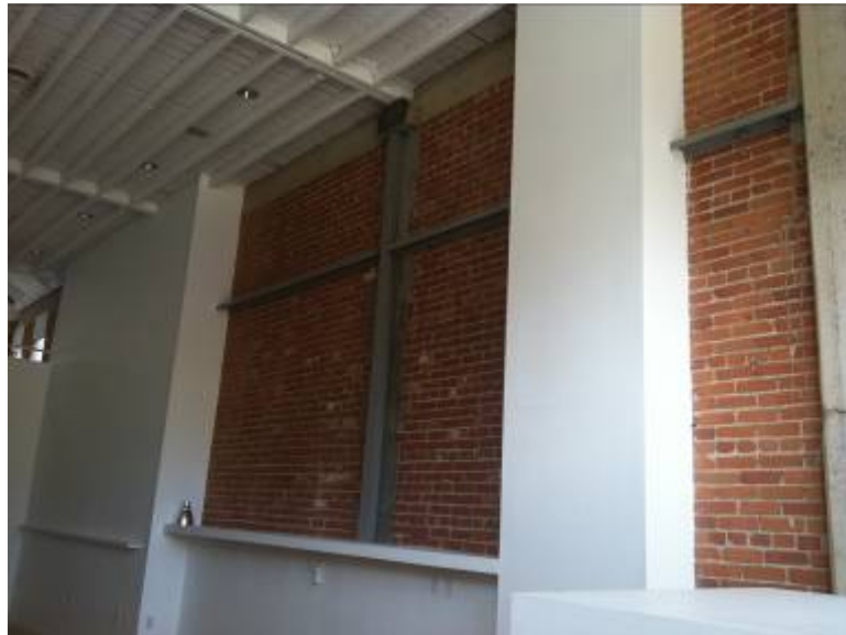
Photo 2: Interior View: Supplemental Gravity Supporting Steel Elements
