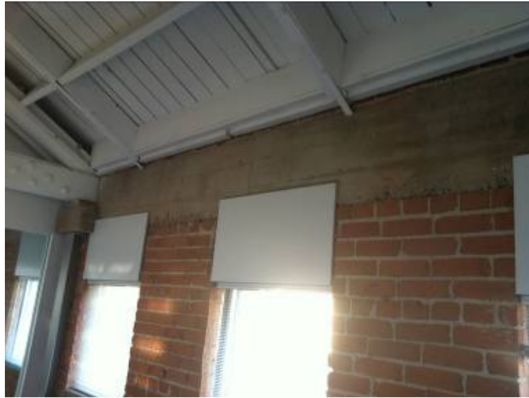
Photo 3: URM Wall to Roof Framing Connections
