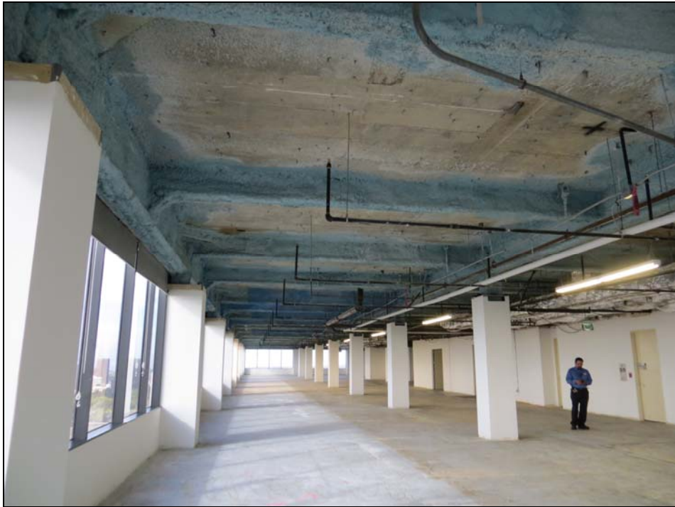
Photo 3 – Typical Floor Framing
