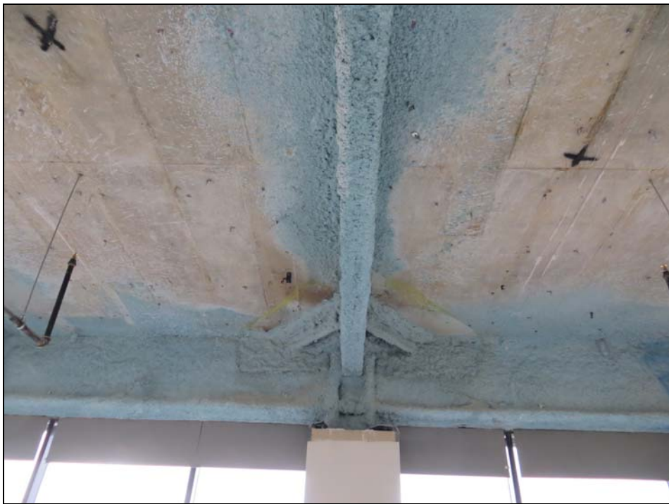
Photo 4 – Typical Beam-to-Column Moment Connection
