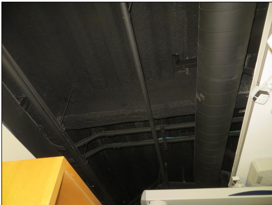
Photo 4 – Typical Steel Framing in Office Floor
