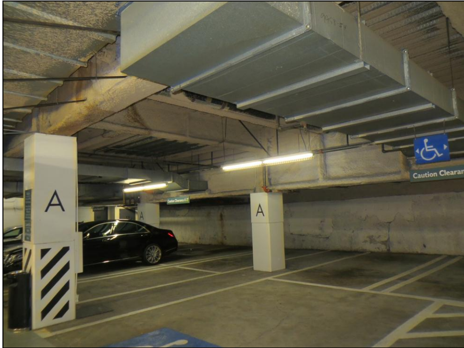
Photo 3 – Steel Framing in Subterranean Level
