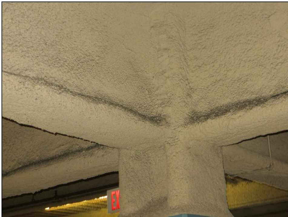
Photo 6 – Typical Welded Moment Connection
