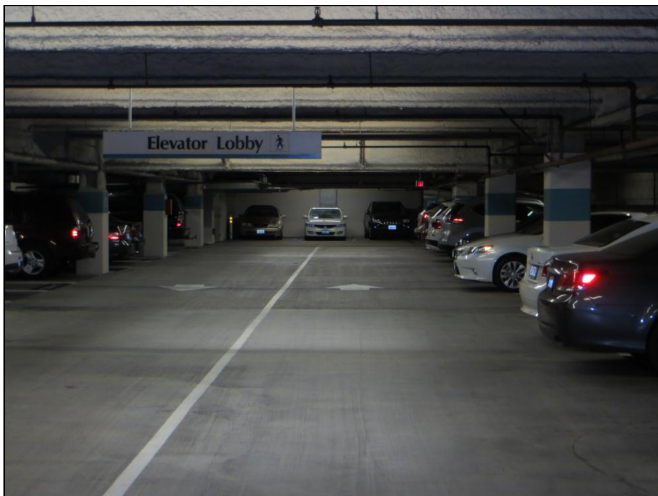
Photo 4 – Typical Steel Framing at Parking Level
