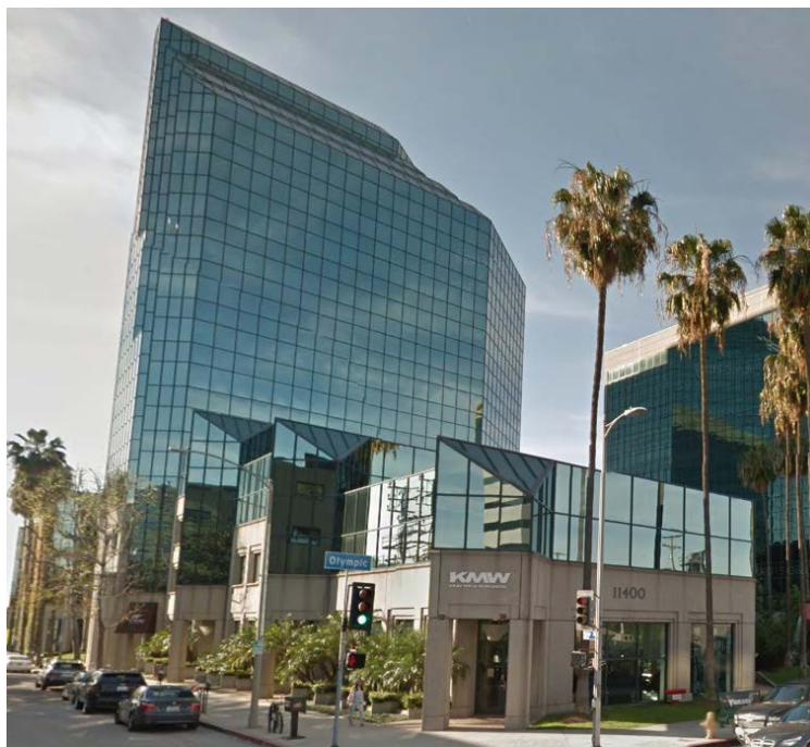
Figure 1 – Northeast elevation of 11400 W. Olympic Boulevard, Los Angeles, CA.
