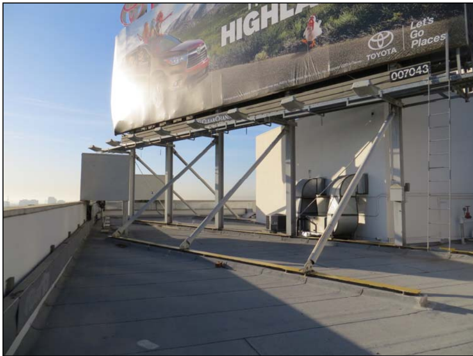
Photo 4 – Bracing of Billboard Frame on Roof
