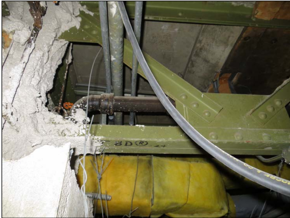
Photo 3 – Typical Steel Truss to Column Connection
