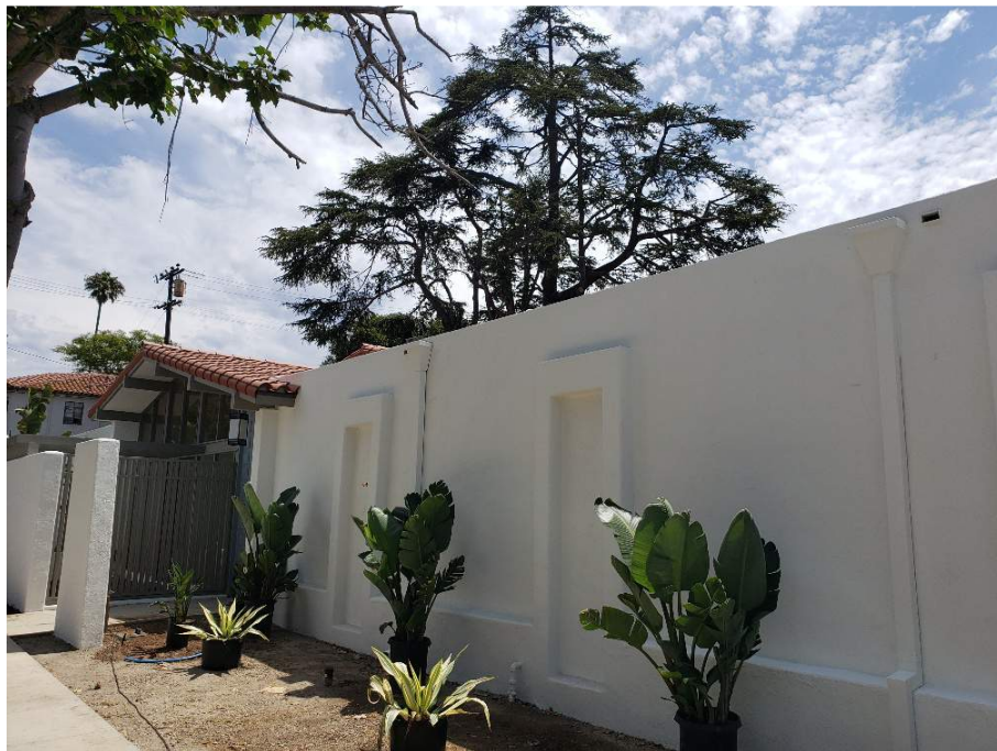
Figure 4 – Northwest Building Elevation (Front Main Entrance - Westernmost Corner View)
