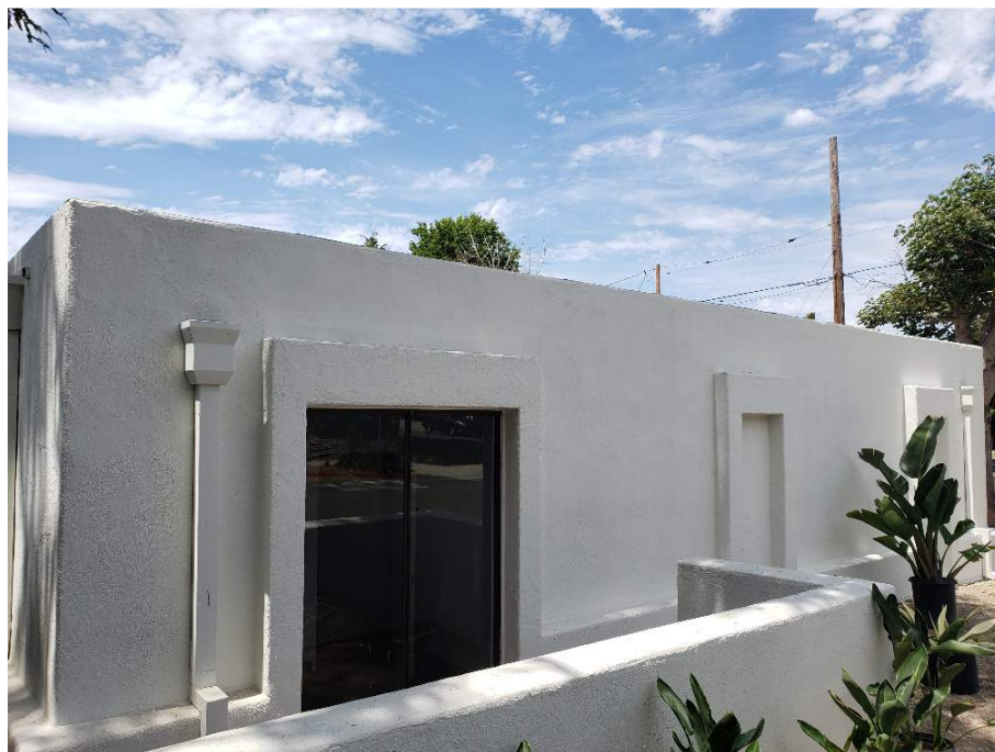
Figure 6 – Northeast Building Elevation (Easternmost Corner View)
