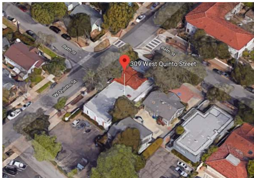
Figure 1 – View of Overall Subject Existing Building Site
