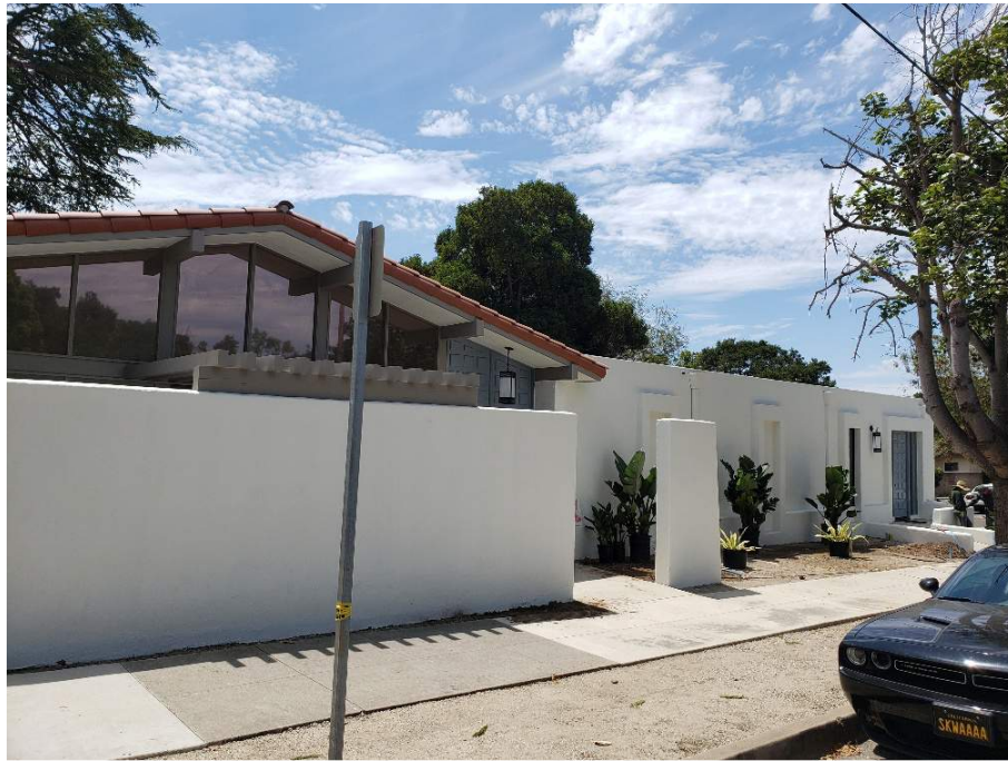
Figure 3 – Northwest Building Elevation (Front Main Entrance - Northernmost Corner View)
