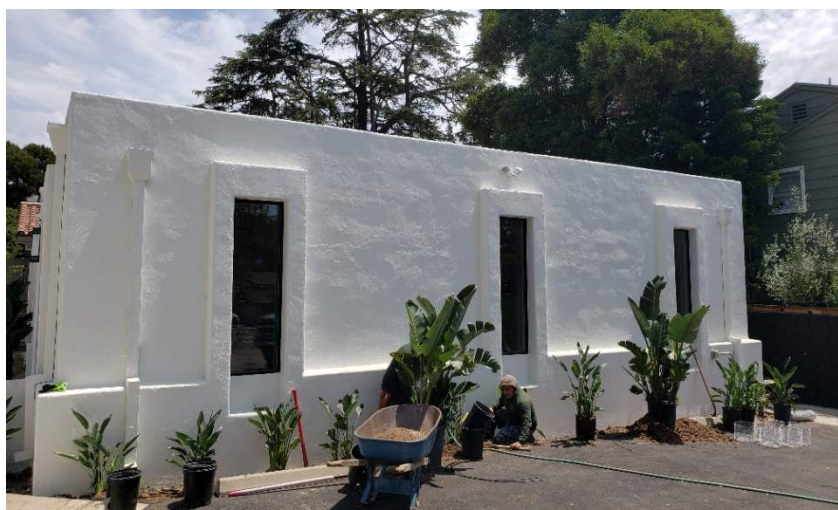
Figure 2 – Southwest Building Elevation (View from Main Parking Lot)
