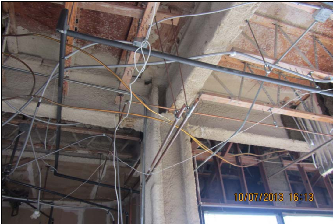
Photo 3 – Typical Steel Framing
