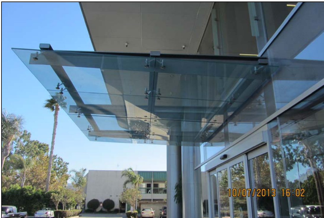
Photo 4 – Canopy at Building Entrance
