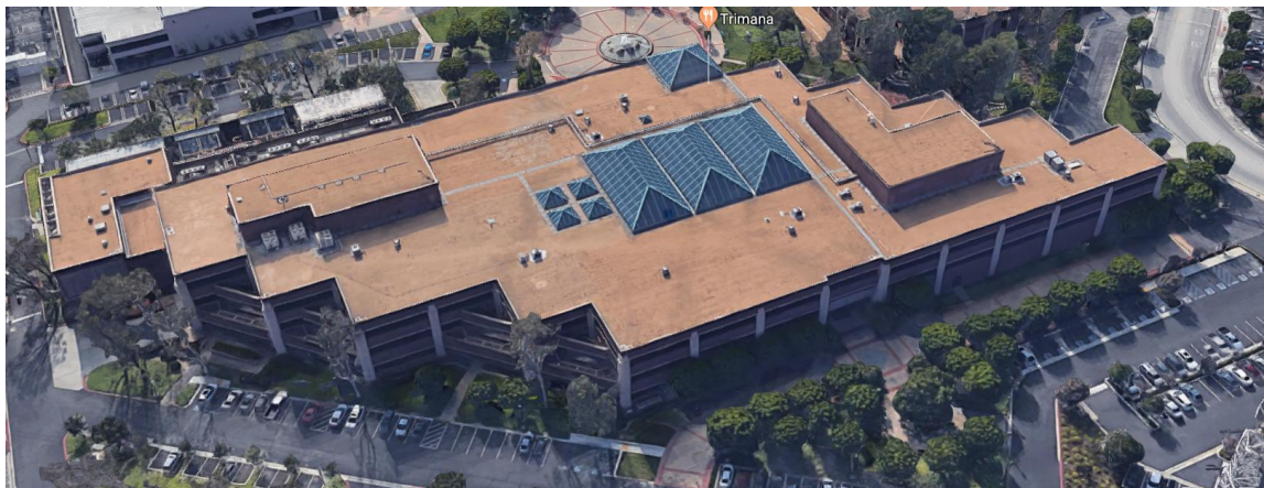
Figure 1 – Overall Building View
