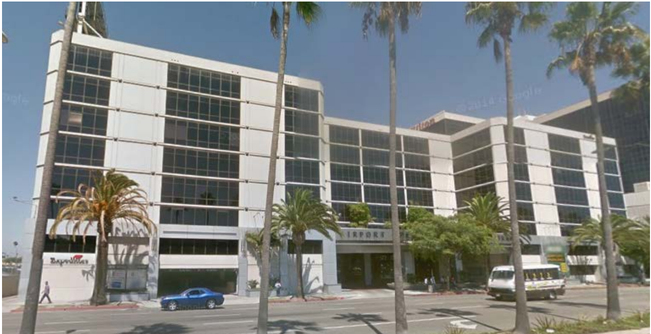
Figure 1 – 5757-5767 W. Century Blvd, Los Angeles, CA; Office Building #1 (South Building) South Elevation
