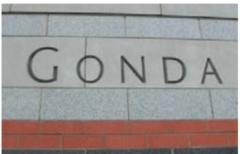
Stone Incised Building Sign
