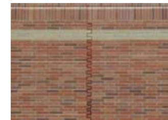
Brick Control Joint
