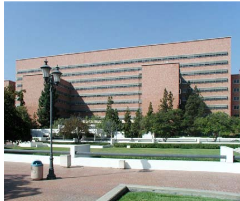
CHS South Tower
