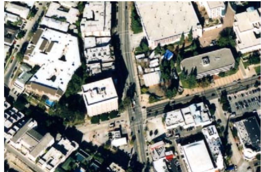
Aerial View of Bridge Zone
