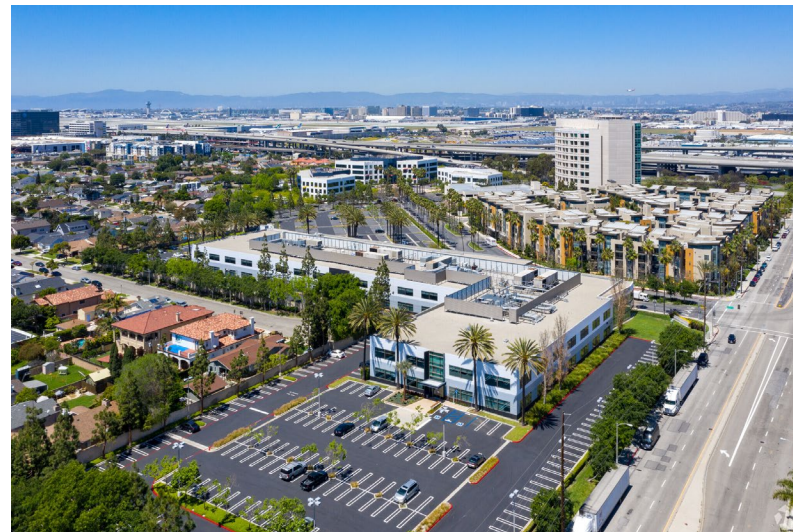
View northwest: south and east facades
