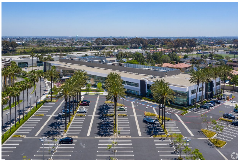
View southeast: north and west facades
